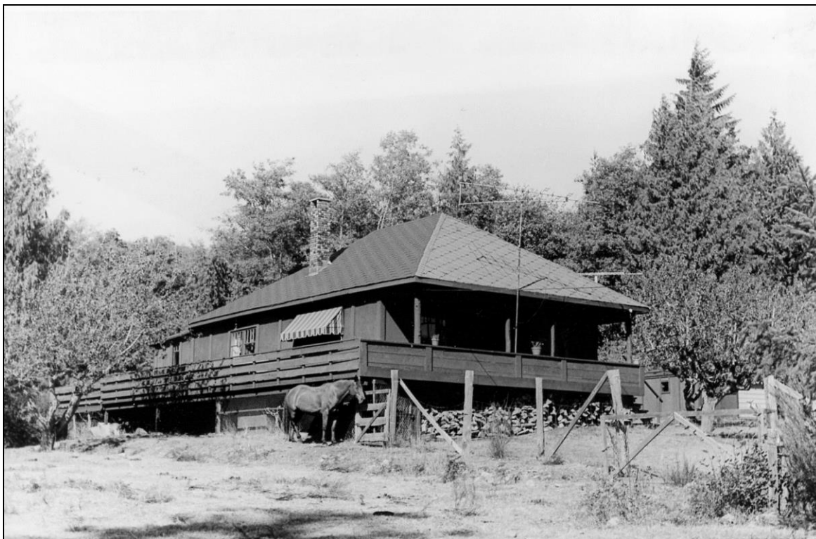
Seaton House, 1984. SRHS #4958
