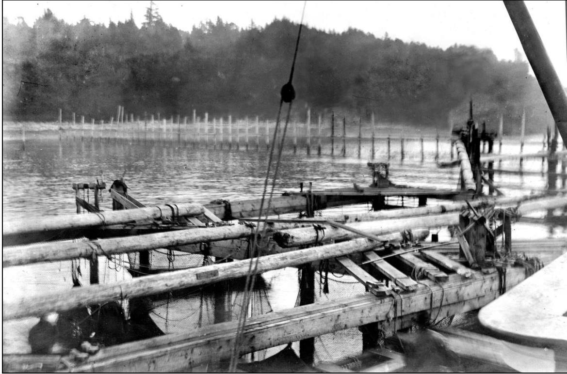
Fish Trap at Otter Point prior to 1920. SRHS #447
