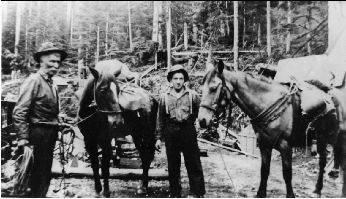
During the Great Depression of the 1930s, construction of the West Coast Road between Grant Road and Tugwell Creek was undertaken by men at the Otter Point Relief Camp. In this scene John Foyer, left, and Bill Witty, right are bringing supplies to the workers along the trail from Sooke to Otter Point. SRHS #3073
