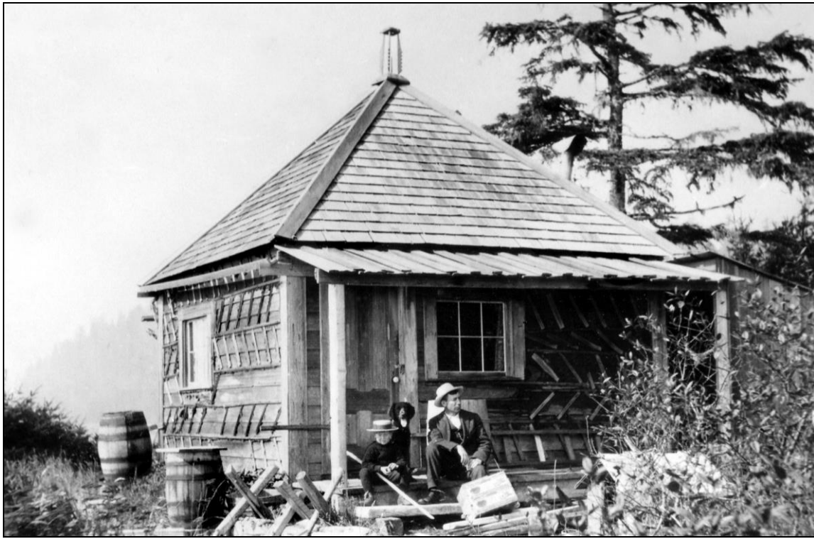
Telegraph linesman's hut along the West Coast Lifesaving Trail near Jordan River. This picture was supplied by Derek Todd of the J. H. Todd fish trap family and was photographed on Sunday, June 5, 1904. The identities of the people in this photo are unknown, but linesman John MacVicar occupied the hut from 1908 onwards. SRHS #3910.
