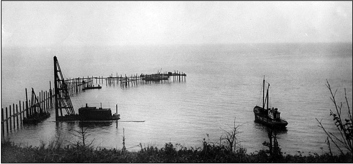
The Otter Point Fish Trap showing how the fir pilings were installed to form the structure of the trap. SRHS #478
