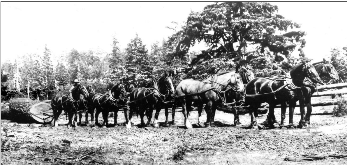
Gordon and Vogel Logging Company. A horse team showed pulling a "sniped" log. Sniping meant cutting the front of the log at an angle to make pulling easier. Reg Clark is the teamster. SRHS #1137
