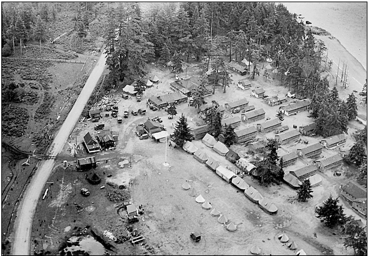
1942 aerial view of the Otter Point Army Camp looking east. The cedar fence at top left was built by Joe Poirier. Present day Carpenter Road is located at the top left and the Olympic View Home Park occupies much of the area in the centre of the picture. This photo came from a collection presented to the Sooke Region Museum by Peter Clegg. SRHS #6908
