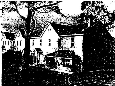
Exterior of Officers' Mess showing attic window.
