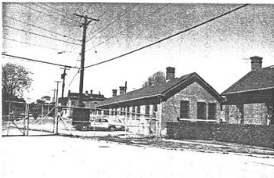
3 Building 1070, rear (south) and end (east) elevations; building no. 1068 is visible at left, no. 1071 stands at right. ( Edward Mills, AHB, Parks, 1989. )
