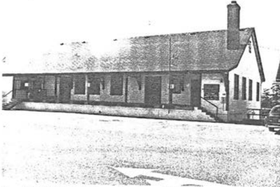
2 Building 1031, main (north) and end (west) elevations. ( Ian Doull, AHB, Parks, 1989. )
