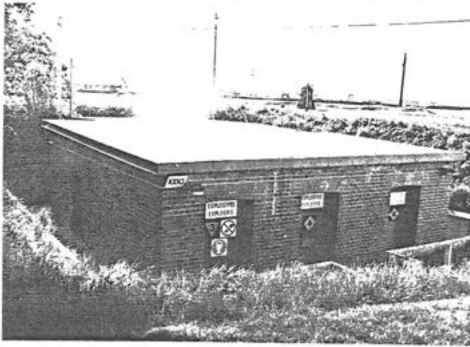
2 Building 1030, main (west) elevation. ( Ian Doull, AHB, Parks, 1989. )
