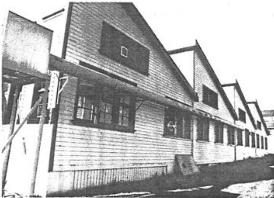
3 Building 1045, north elevation. (Edward Mills, AHB, Parks, 1989.)
