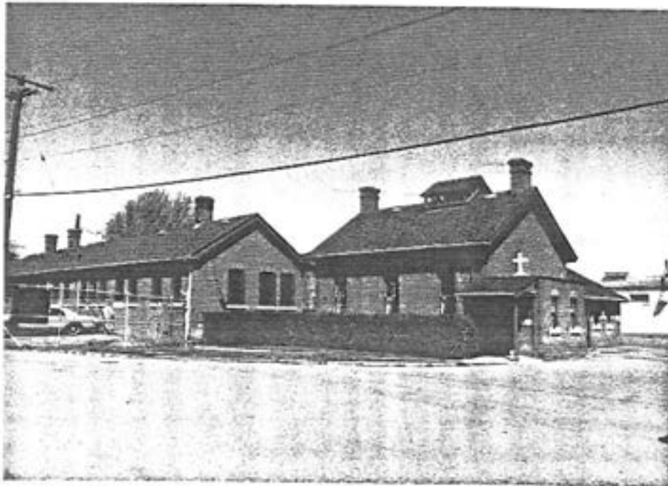
3 Building 1071, south and east elevations. ( Edward Mills, AHB, Parks, 1989. )
