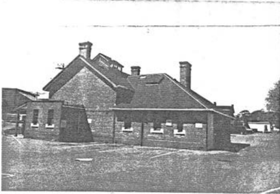
2 Building 1071, eastern elevation. ( Edward Mills, AHB, Parks, 1989. )
