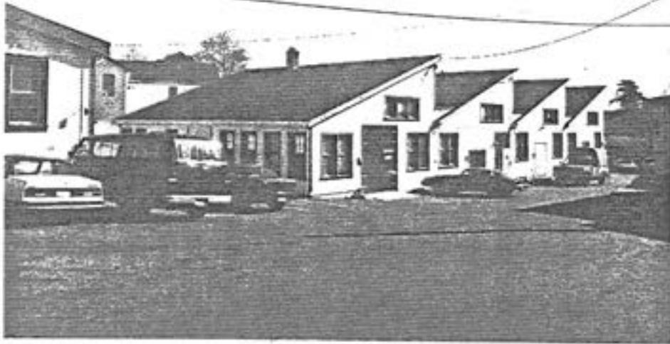
2 Building 1045, end (west) and side (south) elevations; building 1044 stands at left. (Edward Mills, AHB, Parks, 1989.)
