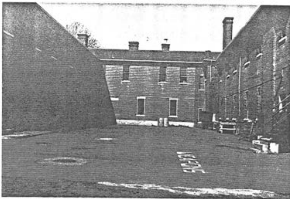
4 Building 1075, connecting wing, looking west. ( Ian Doull, AHB, Parks, 1989. )
