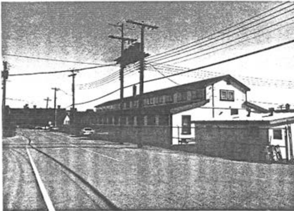
3 Building 1044, end (south) and side (west) elevations. ( Edward Mills, AHB, Parks, 1989. )
