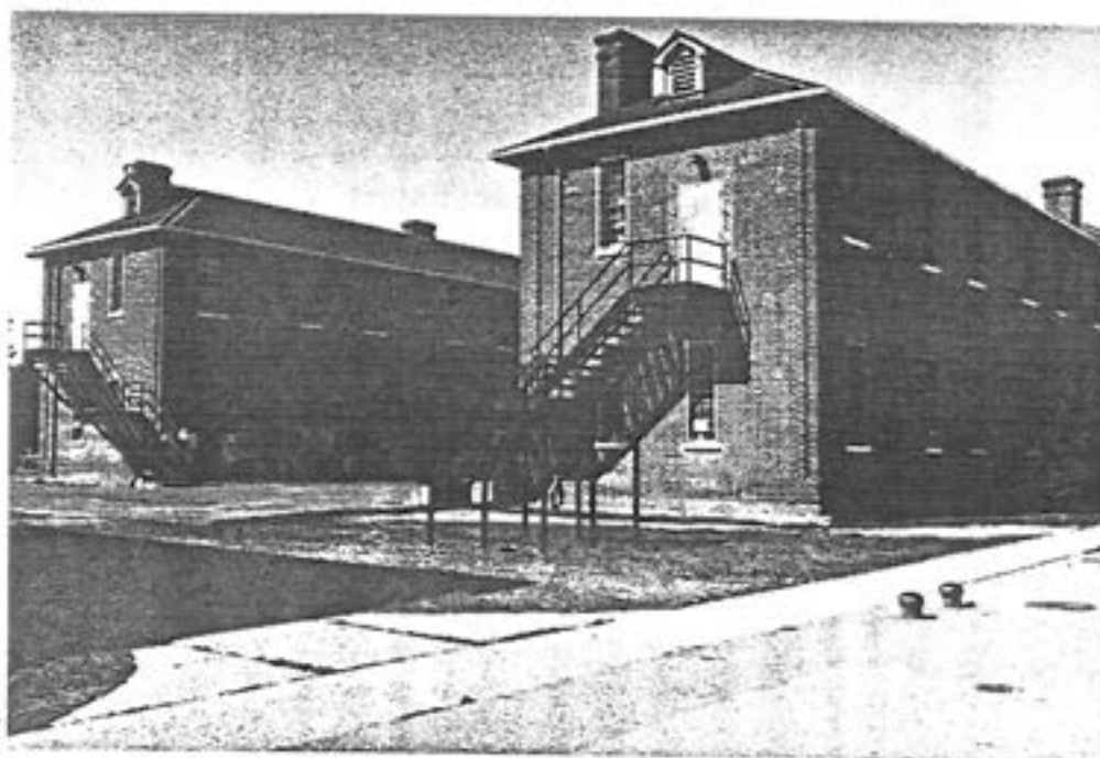
5 Building 1075, end (east) elevations. ( Ian Doull, AHB, Parks, 1989. )
