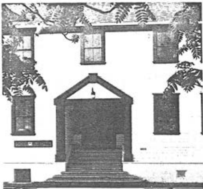
4 Building 1033, main entrance detail. (Ian Doull, AHB, Parks, 1989.)
