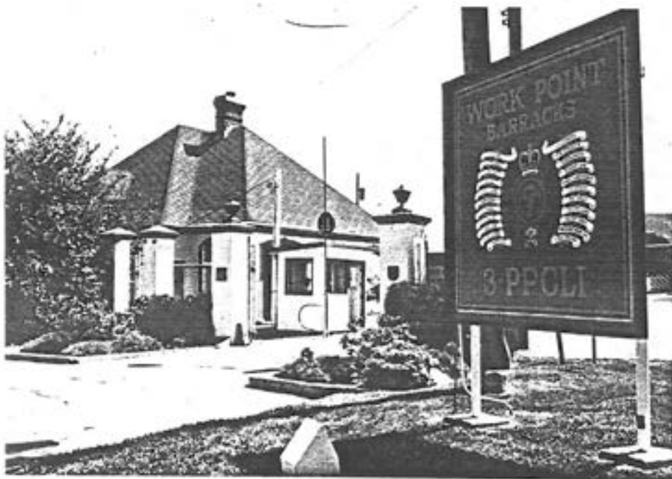
8 Building 1001 and main gateway to Work Point. ( Ian Doull, AHB, Parks, 1989. )
