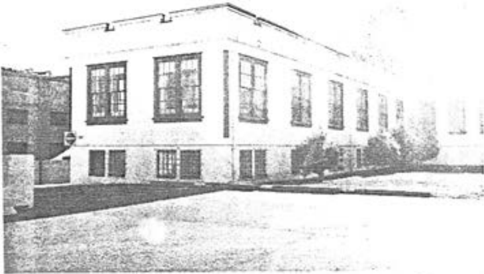
4 Building 1020, western wing, south (side) and west (end) elevations. ( Ian Doull, AHB, Parks, 1989. )
