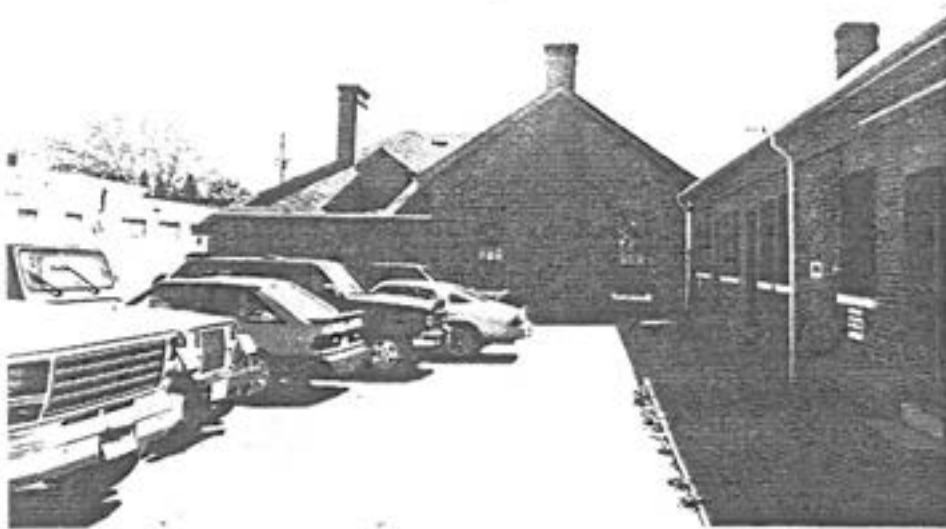
4 Building 1071, west elevation; building 1070 stands at right. ( Edward Mills, AHB, Parks, 1989. )
