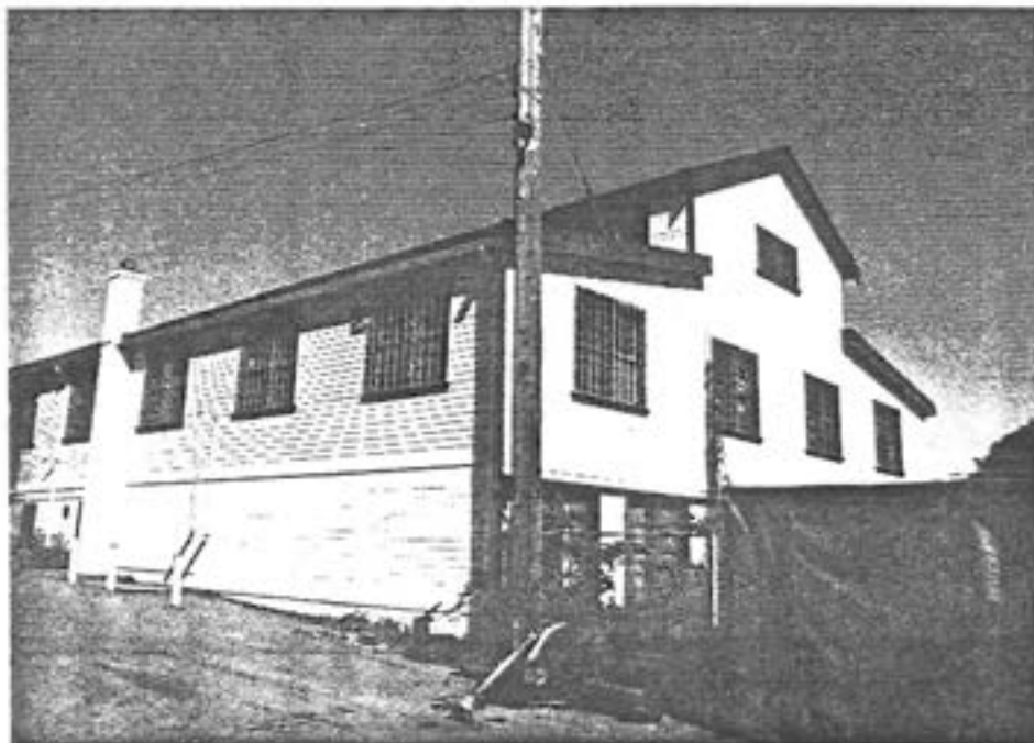
3 Building 1048, end (east) and side (south) elevations. ( Edward Mills, AHB, Parks, 1989. )
