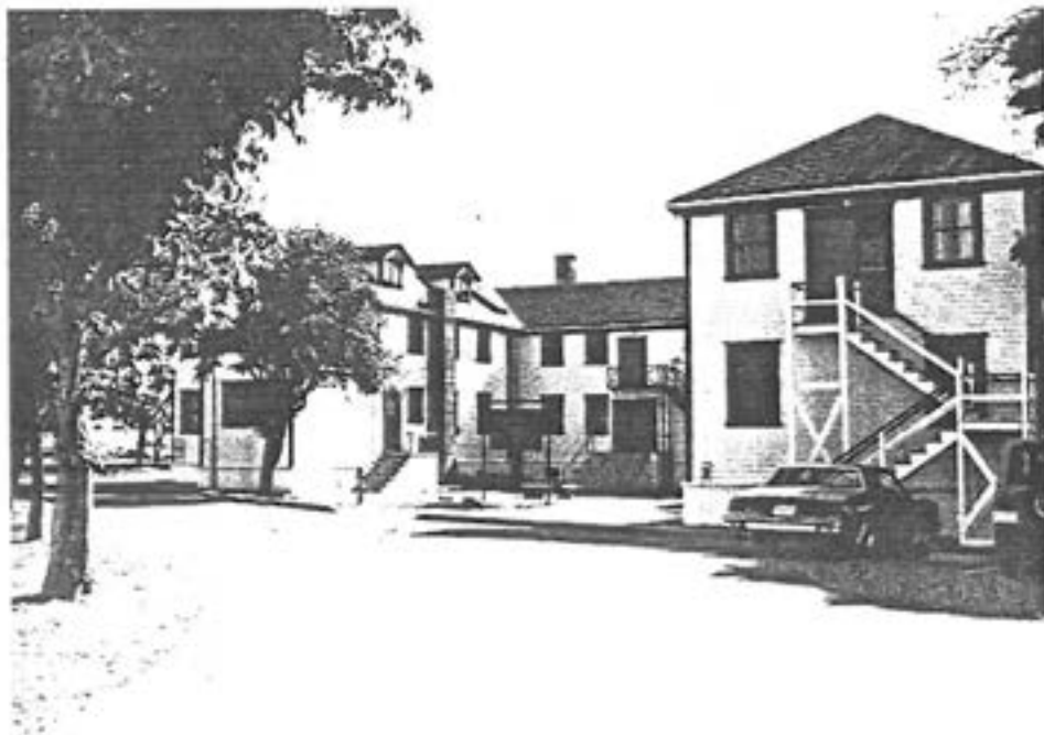
5 Building 1033, original section at left, looking northeast. (Ian Doull, AHB, Parks, 1989.)
