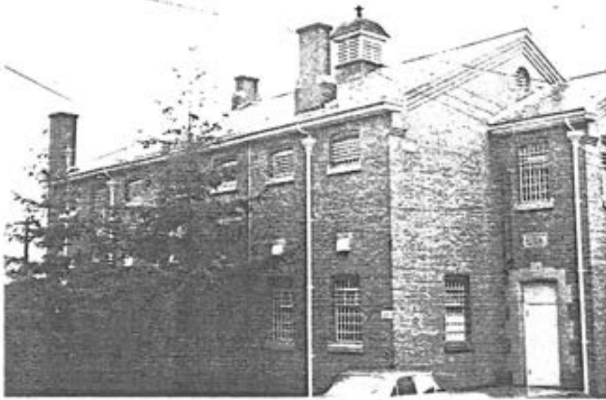
4 Building D26-D27, former Dockyard prison, constructed 1899. ( CIHB, Parks, 1971. )
