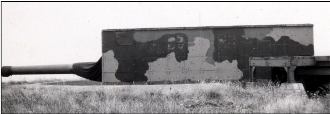
A C Mk 6A mounting in place at Albert Head battery. The Canadian version of the design replaced the open barbette style mounting with a slab-like gun house. 15 Field Regiment, RCA, Archives.
