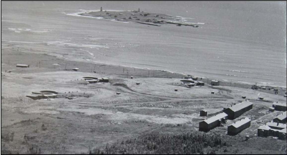
Devils Battery looking seaward on 13 August 1941. The island is at the top, with the three gun positions in the centre of the photo. The emplacements are empty as the guns and mountings have not yet arrived. The administrative area is the group of buildings to the lower right. This photo shows clearly the proximity to the sea and the low-lying nature of the battery. Devils Battery Fort Record Book.
