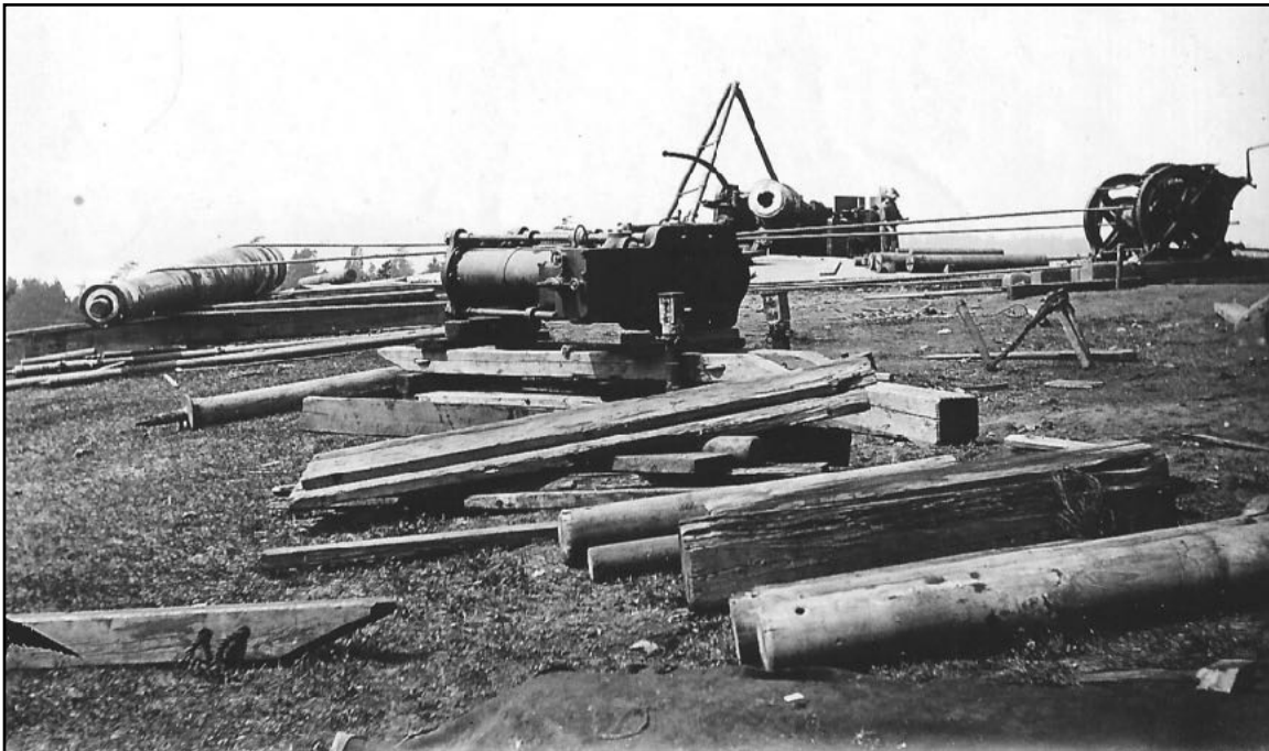
Mounting the guns at Signal Hill, Esquimalt, about 1912. The first gun appears to be basically assembled, with the tripod gun still in place. The second gun barrel is being parbuckled (winched and rolled) up a timber roadway. The timber in the foreground gives an idea of the size needed for the ramp supports and rollers. Notice the complete lack of engines or power machinery. Fort Rodd Hill via Jack Bates.
