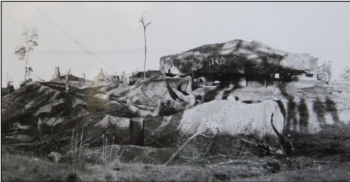
A 9.2-inch gun on a Mk 5 mounting camouflaged with wire and chicken feathers at Albert Head early in the Second World War. Note the shadows of the men on the right. LAC Albert Head Fort Record Book.
