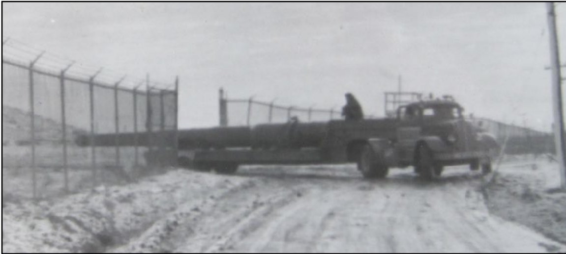
The last gun barrel leaves Devils Battery in November 1954 on a civilian tractor-trailer. The weight was approximately 31 tons. The trailer was 23 feet (~7 m) long, and the overhang was 14 feet (~4.3 m). Devils Battery Fort Record Book,
