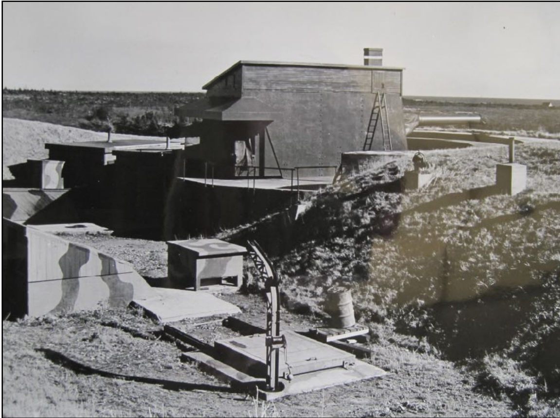
9.2-inch Mk 10 gun on Mk 7 mounting at Devils Battery in Halifax during the Second World War. The gun is camouflaged as a house. The entrance and hoist to the magazine is in the foreground. Devils Battery Fort Record Book.
