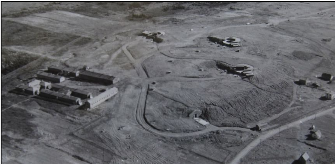
An aerial view of Devils Battery on 30 October 1941. The sea and the main arc of fire is to the upper right. The entrance to the tunnels and engine room is in the foreground, and the line of the tunnels can be seen by tracing the escape hatches. The left and right gun emplacements have guns mounted, but the centre emplacement is empty as its mounting had not yet arrived. The buildings to the left are the administrative area. The battery observation post is out of the photo to the left. Devils Battery Fort Record Book.
