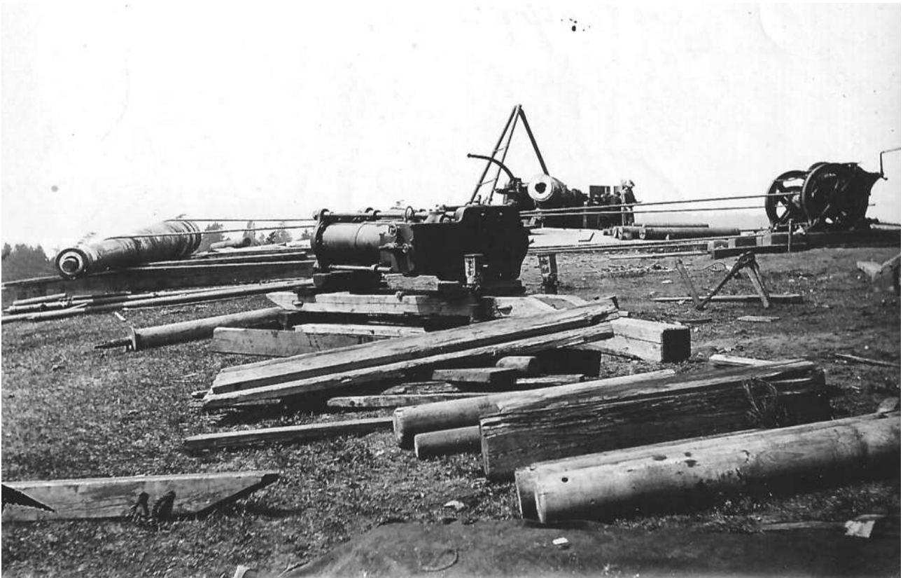
'Parbuckling' a 28 ton 9.2-inch BL barrel into position at Signal Hill Battery using a winch, note: the recoil accumulator is on a wooden sleigh in the foreground. (Rodd Hill National Memorial archive)
