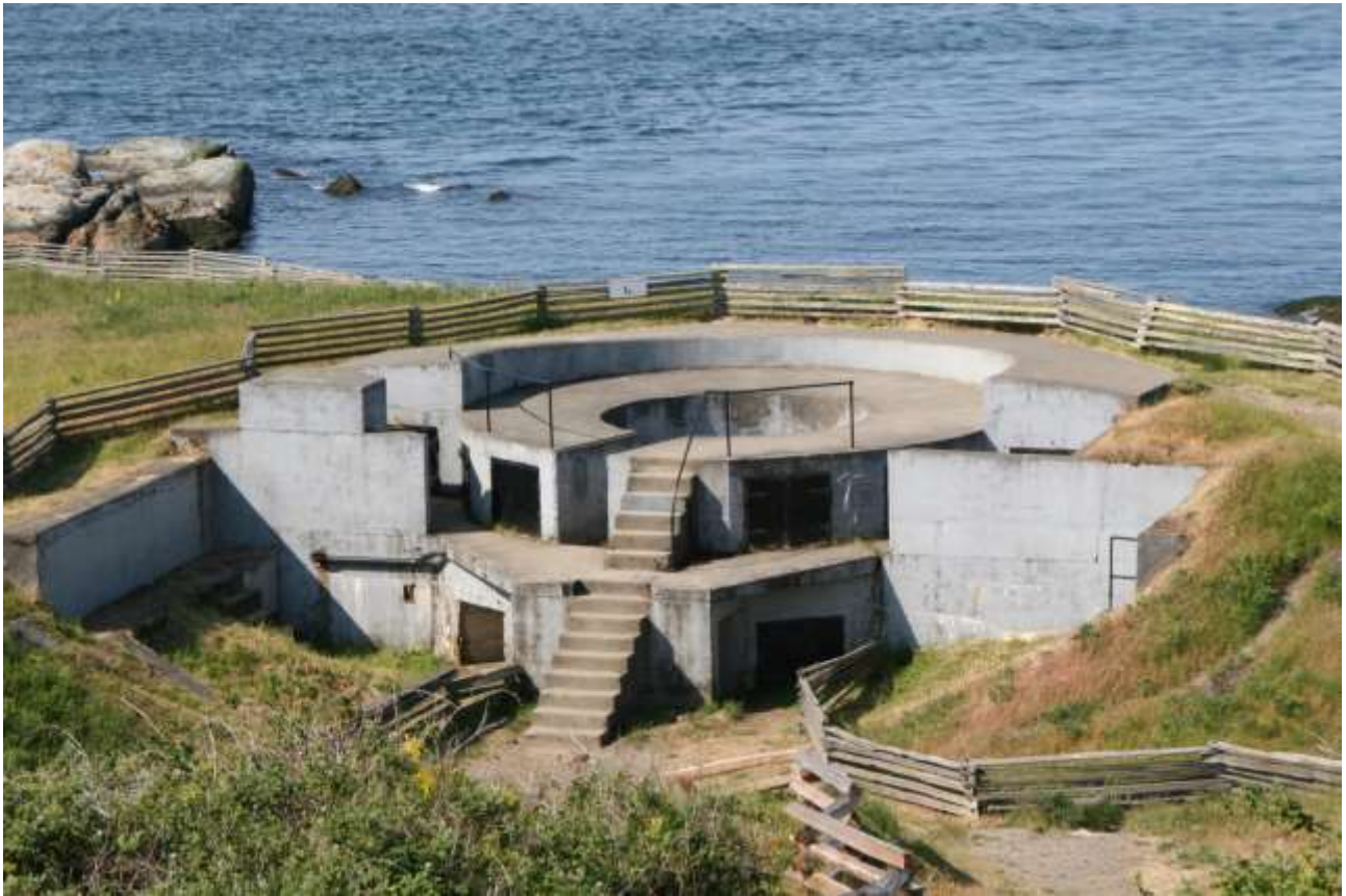
Macaulay Point Battery - 6-inch gun position originally a disappearing mounting with a 6-inch BL CP emplacement built within the pit
