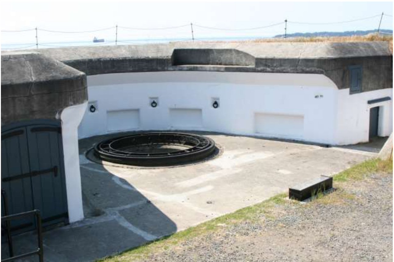
Rodd Hill - Two Gun Battery. 6-inch BL Disappearing Gun pit
