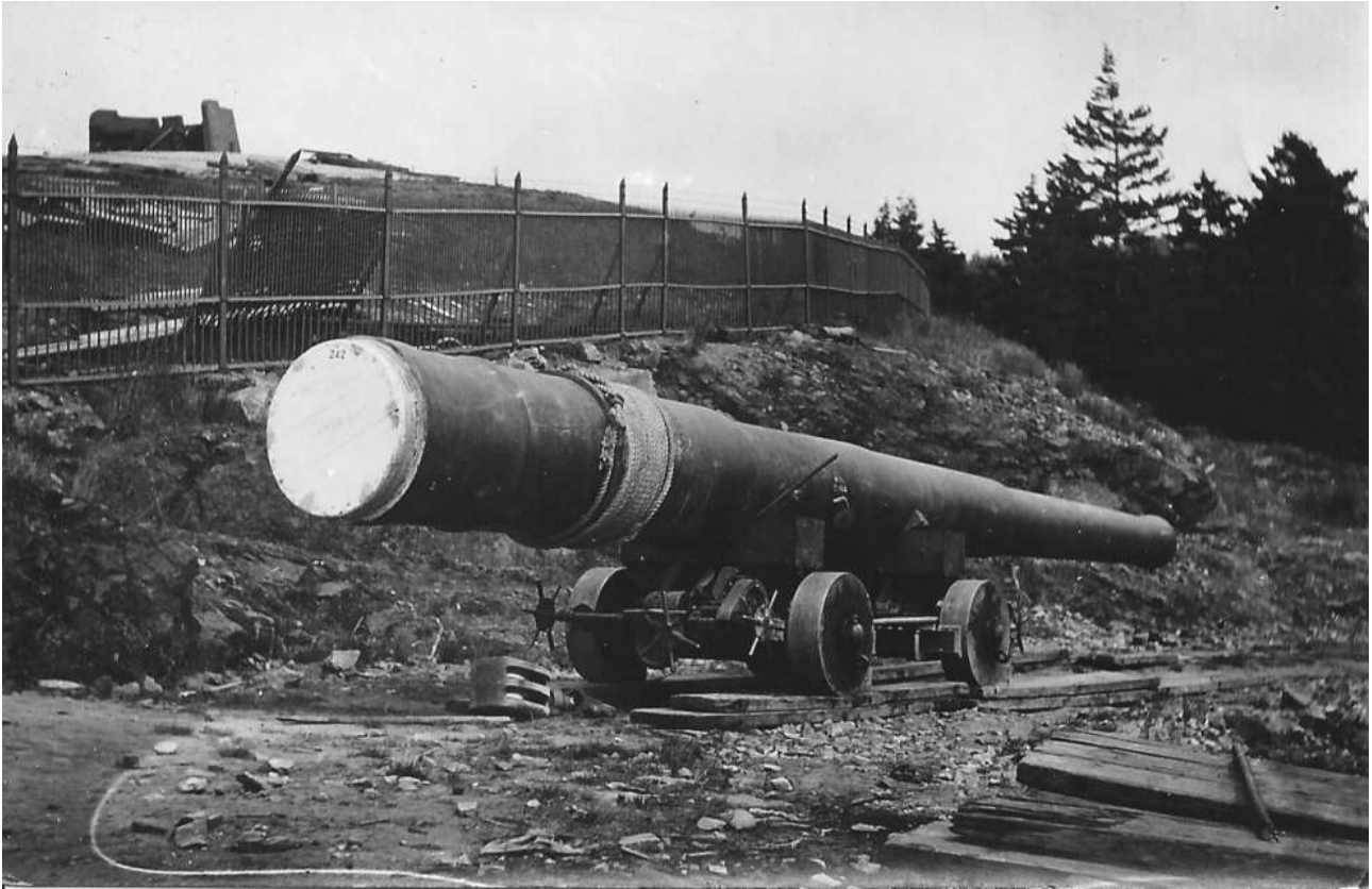
9.2-inch BL gun barrel being moved up Signal Hill using a 30 ton Gun Drug (Rodd Hill National Memorial archive)
