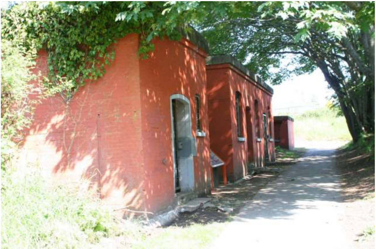
Macaulay Point Battery - Store, Smiths & Fitters Shops & Small Arms magazine
