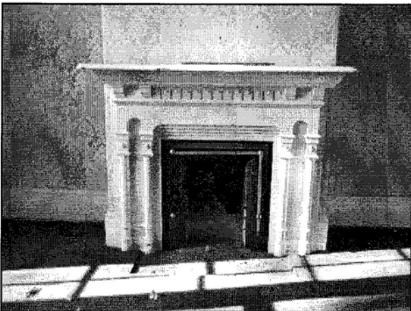
Fireplace with historic wallpaper above. May 11, 2003
