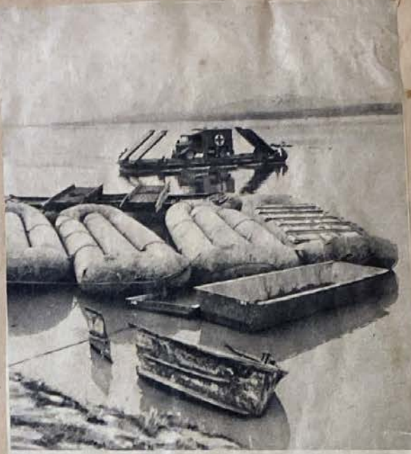
A FERRY CARRIES an ambulance across this estuary, and the pontoons in the foreground formed part of a bridge the floods broke up. The Pats have shown engineering skill in meeting road and bridge problems.
