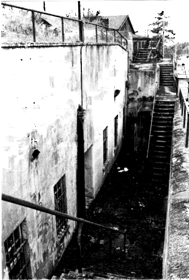
6 Signal Hill emplacement, view across magazine area toward western gun position. ( CIHB, Parks, 1974. )
