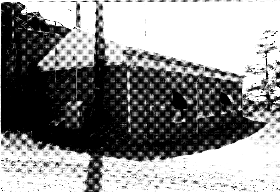
8 Signal Hill building no. 546, main and side (east) elevations. (Ian Doull, AHB, Parks, 1989.)
