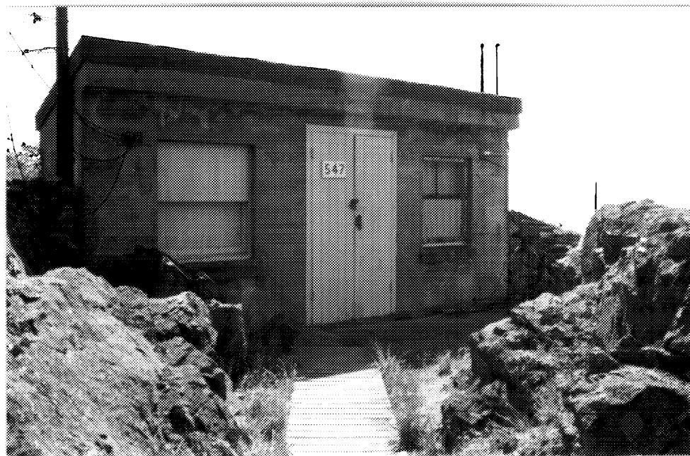
10 Building 547, main elevation. ( Ian Doull, AHB, Parks, 1989. )
