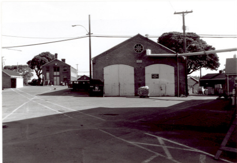
7 Building D60, southern elevation; buildings D69, D68 to left, D56, D55 to right. ( Ian Doull, AHB, Parks, 1989. )
