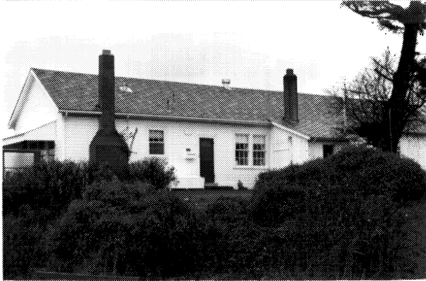
4 Building D106, rear (eastern) elevation. (CIHB, Parks, 1976.)
