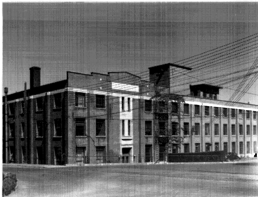
30 Building D192-D192B, southern elevation, 1954. ( NA, PA-176352. )
