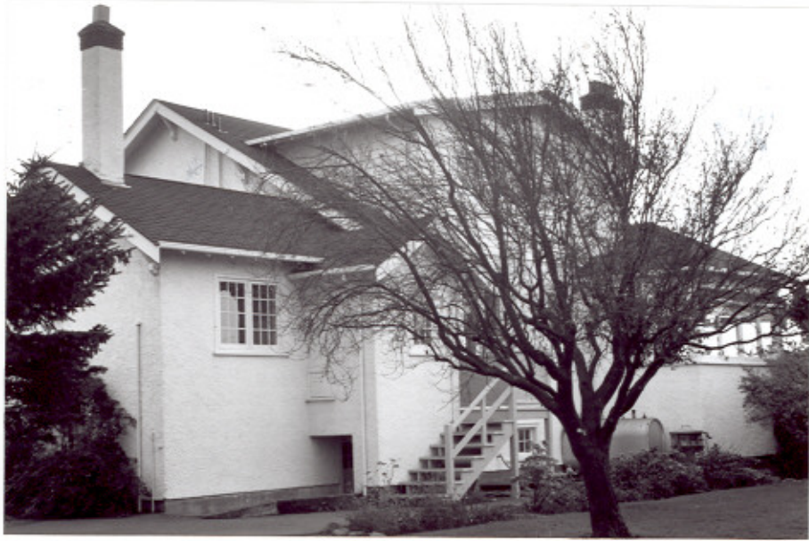
4 Building D194, western elevation. ( CIHB, Parks, 1986. )
