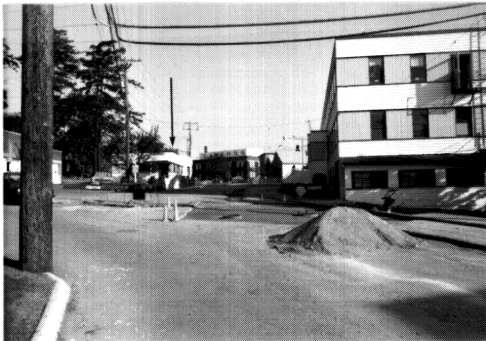
6 Building D37, setting, looking northwest on Hospital Road from building D50, at right. (Ian Doull, AHB, Parks, 1989.)
