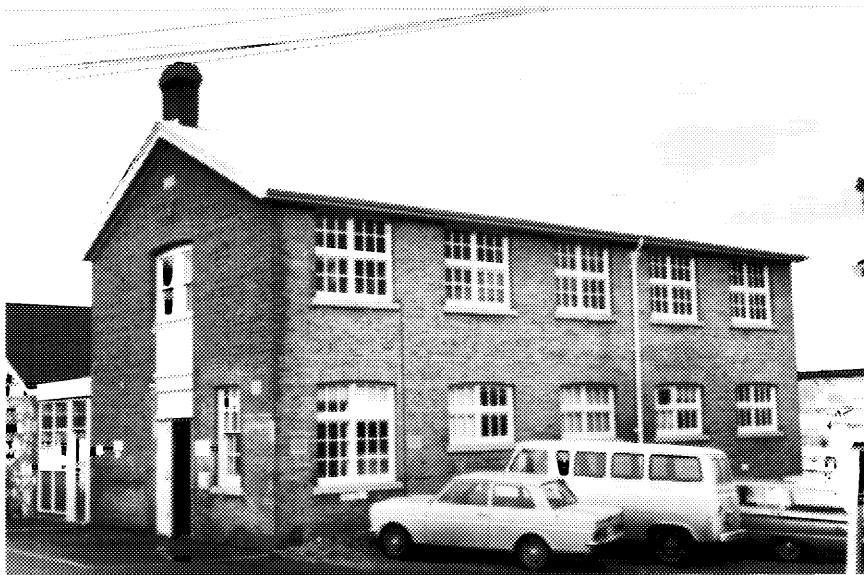
2 Building D63, main (west) and side (south) elevations. ( CIHB, Parks, 1970. )
