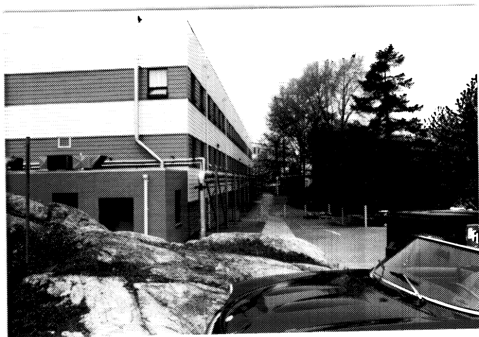
5 Building D49, eastern elevation. (Ian Doull, AHB, Parks, 1989.)
