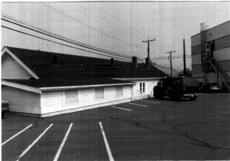
3 Building D188, western (rear) elevation, from raised parade square. ( Ian Doull, AHB, Parks, 1989. )
