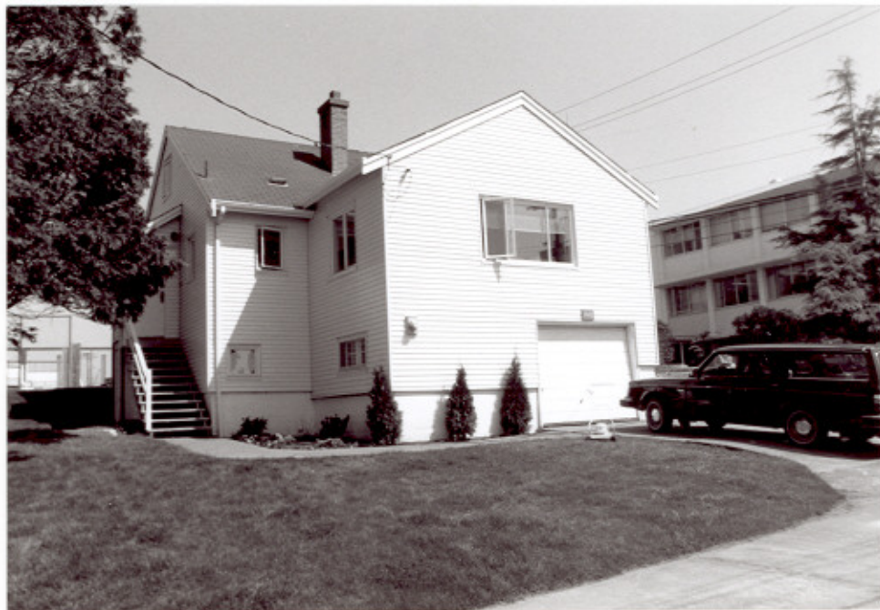
3 Building D198, southern elevation; building D199 stands at right. (Ian Doull, AHB, Parks, 1989.)
