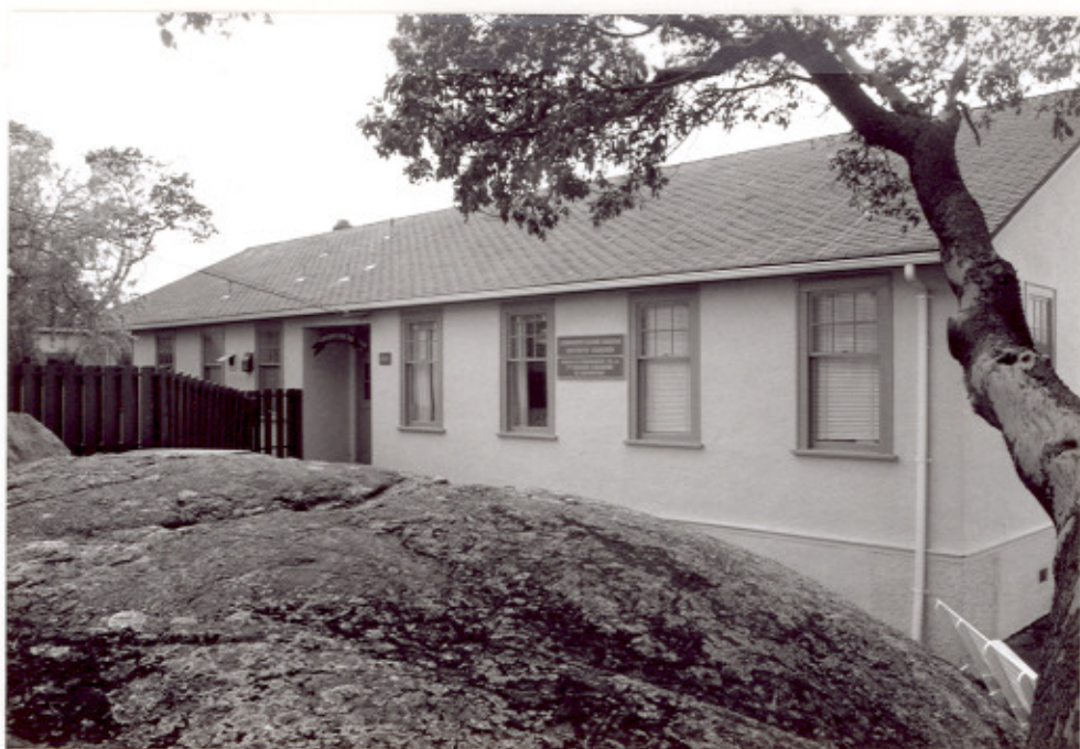
2 Building D66, main (eastern) elevation. ( Ian Doull, AHB, Parks, 1989. )
