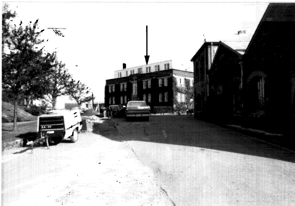
28 Building D70, main (southern) elevation. ( Ian Doull, AHB, Parks, 1989. )
