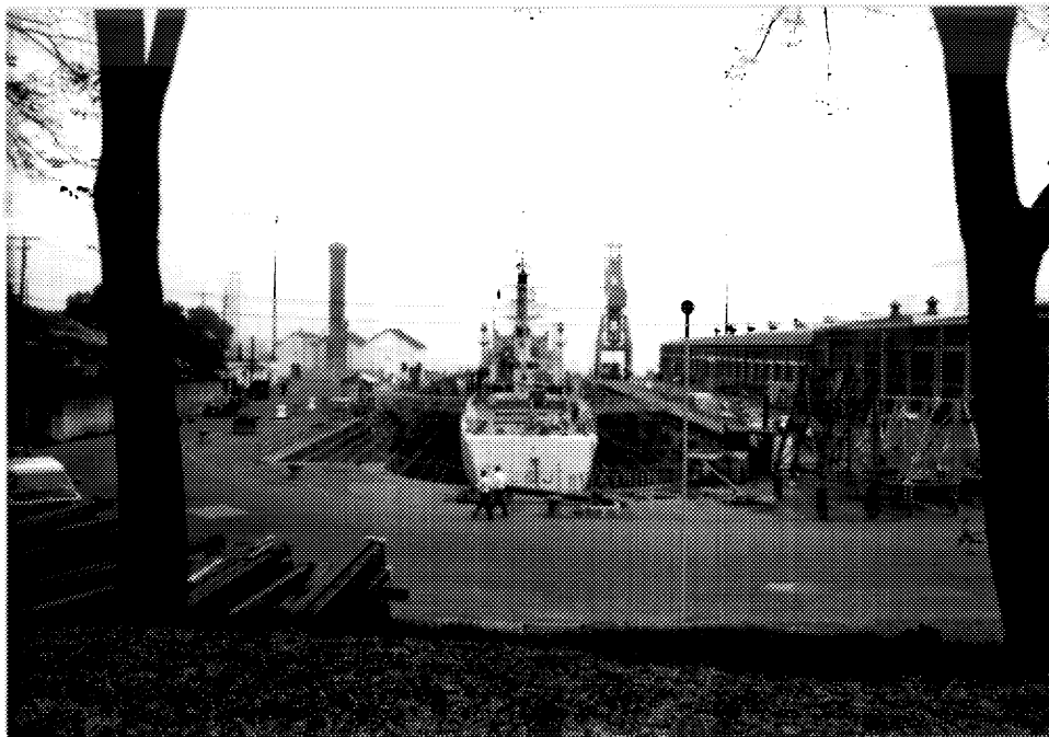
39 Drydock; building D175 at left, D190-D191B-D191 at right. ( Ian Doull, AHB, Parks, 1989. )
