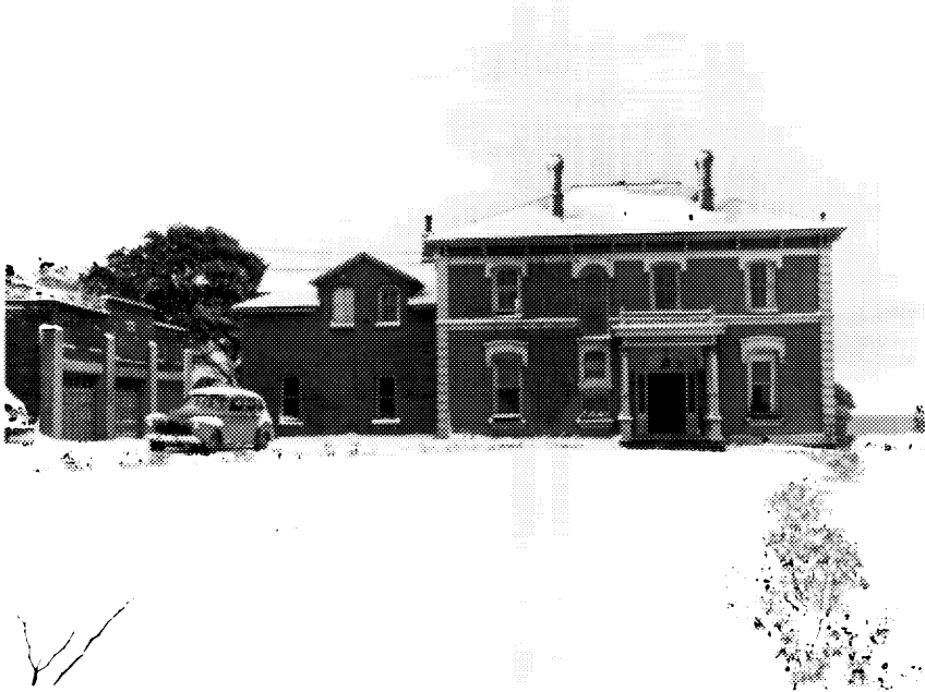
3 Building D101, main elevation, as altered, 1949. ( NA, PA-176370. )
