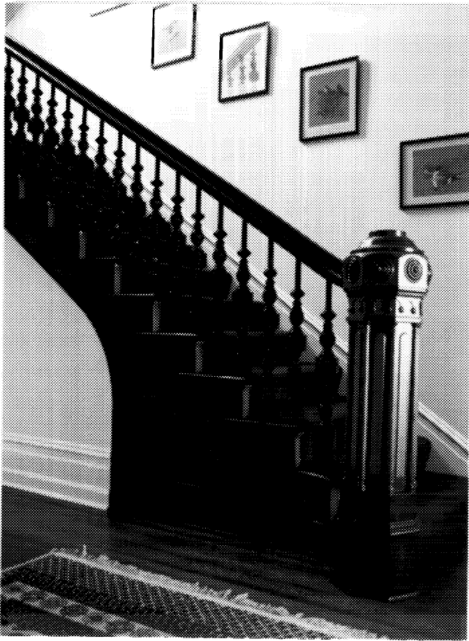
16 Building D101, main staircase, detail. (Ian Doull, AHB, Parks, 1989.)
