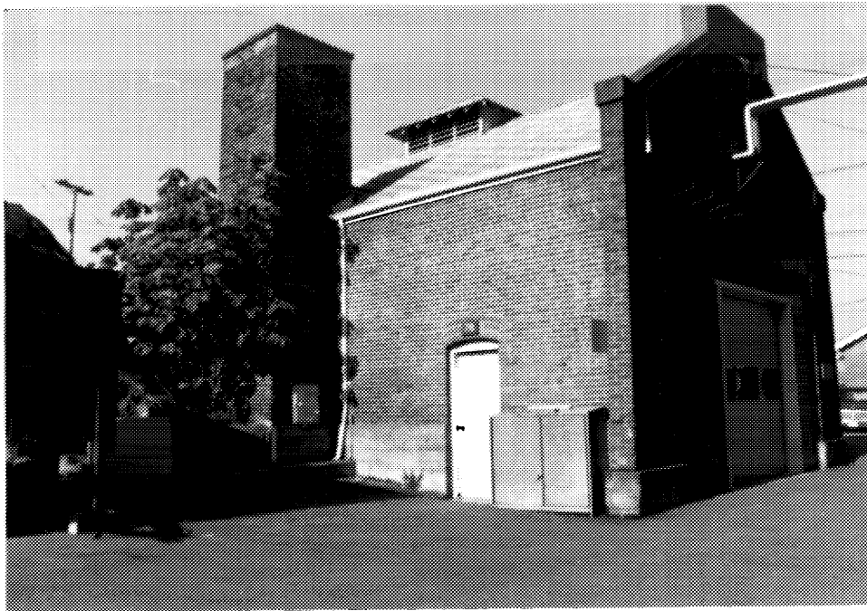
2 Building D78, end (northern) and side (eastern) elevations. ( Ian Doull, AHB, Parks, 1989. )
