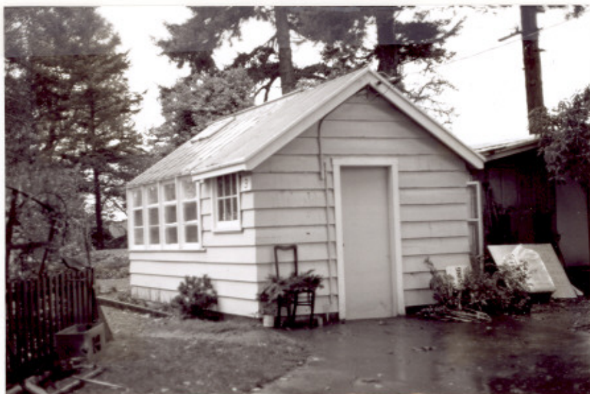
2 Building D3B, side (eastern) and main (northern) elevations. ( CIHB, Parks, 1976. )
