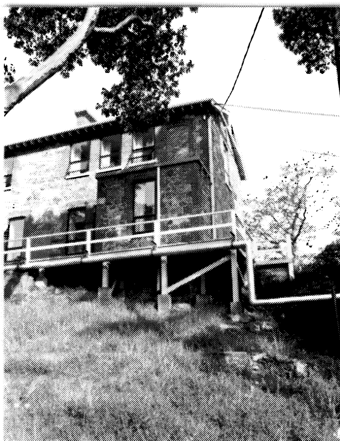
8 Building D38, southeastern corner. ( Ian Doull, AHB, Parks, 1989. )
