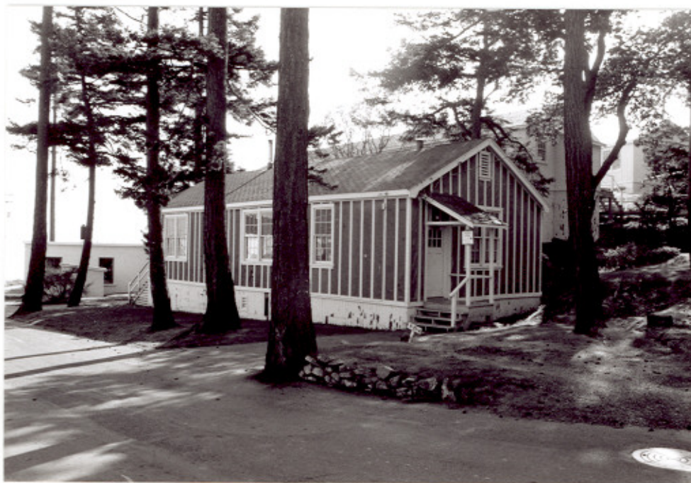
3 Building D244, side (eastern) and rear (northern) elevations. ( Ian Doull, AHB, Parks, 1989. )
