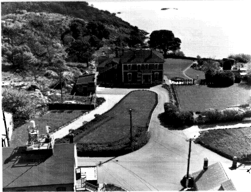
24 Building D101, site details, looking south, 1953. (NA, PA-176381.)
