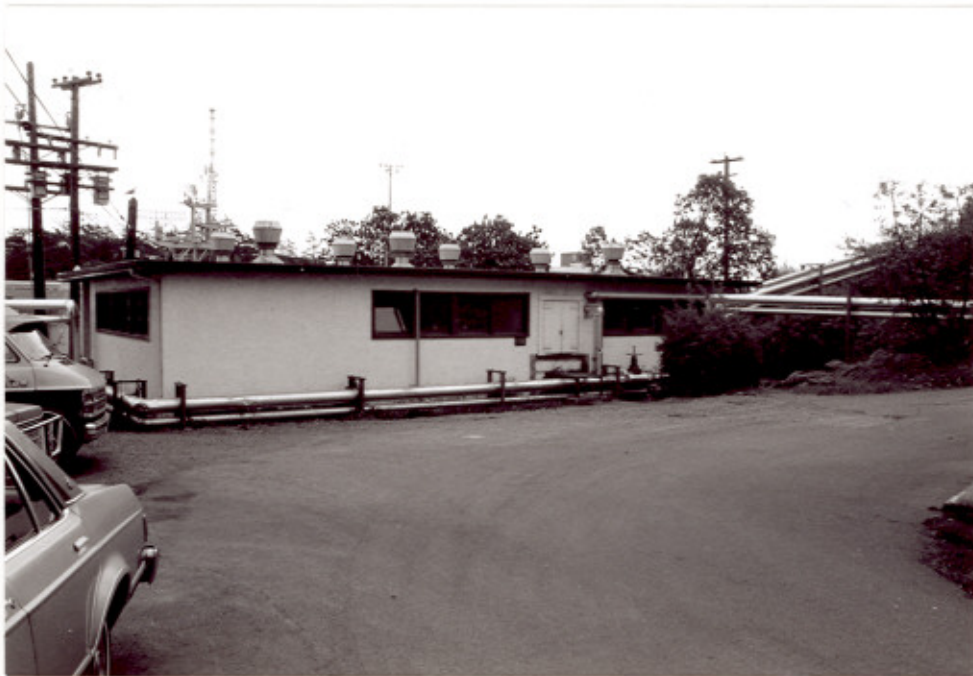
3 Building D172, rear (western) elevation. ( Ian Doull, AHB, Parks, 1989. )
