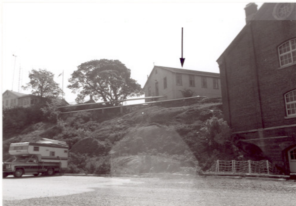
5 Building D66 from vicinity of "A" Jetty; building D71 stands at extreme left, D85 at right. (Ian Doull, AHB, Parks, 1989.)
