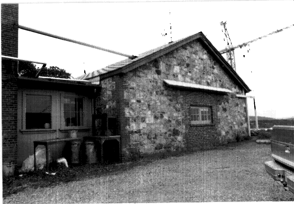
3 Building D64, rear (eastern) elevation. (Ian Doull, AHB, Parks, 1989.)
