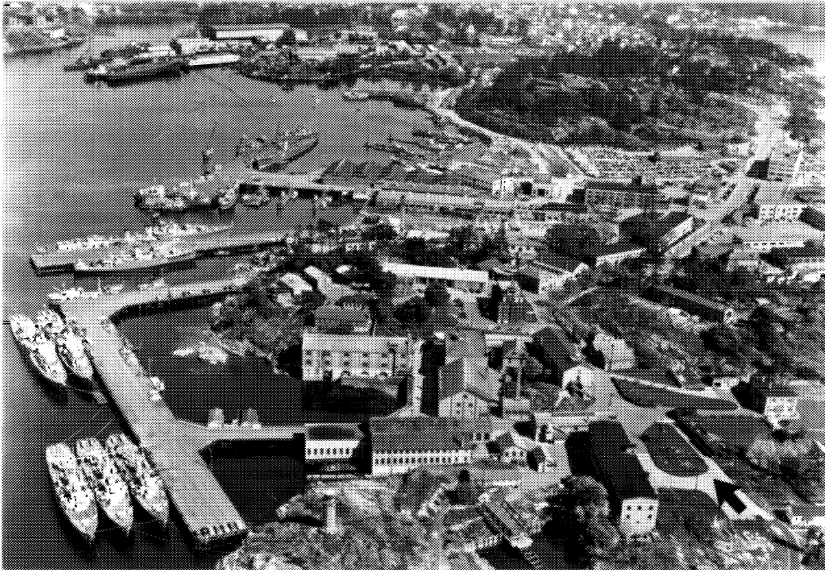
34 Esquimalt Dockyard, looking eastward along Hospital Road (arrow), from its western terminus at Duntze Head, 1953. (NA, PA-169976.)
