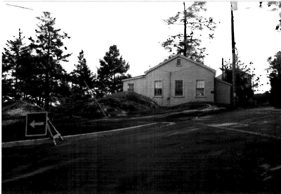
5 Building D217, northern elevation. ( Ian Doull, AHB, Parks, 1989. )
