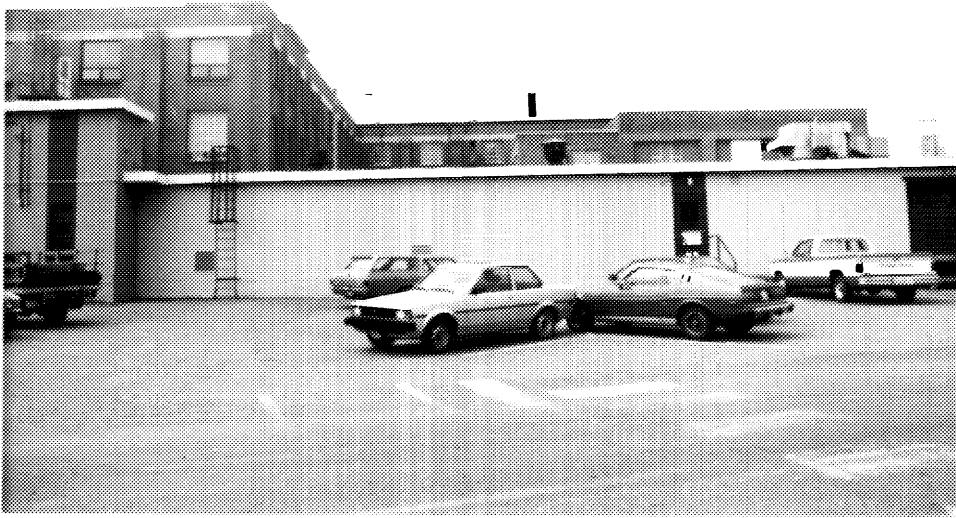
2 Building D139, eastern elevation, with the D192 grouping in the background. (Ian Doull, AHB, Parks, 1989.)
