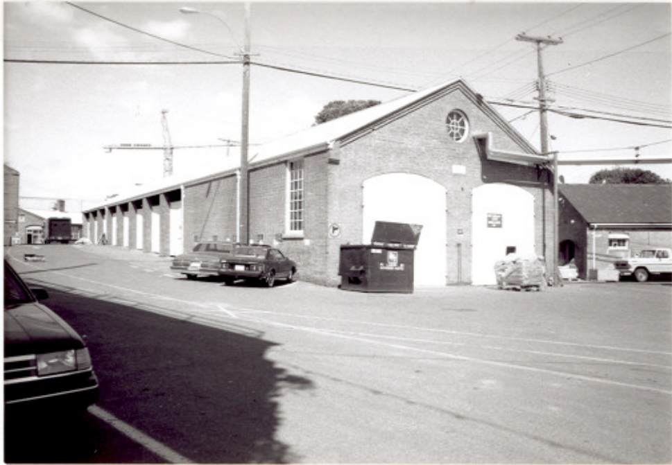
2 Building D60, end (southern) and side (western) elevations; building D55 stands at right. ( Ian Doull, AHB, Parks, 1989. )
