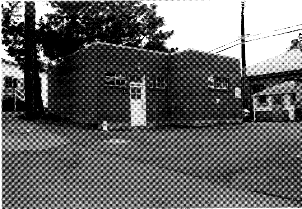
2 Building D53, main (northern) elevation; buildings D178 and D51 to left and right. ( Ian Doull, AHB, Parks, 1989. )
