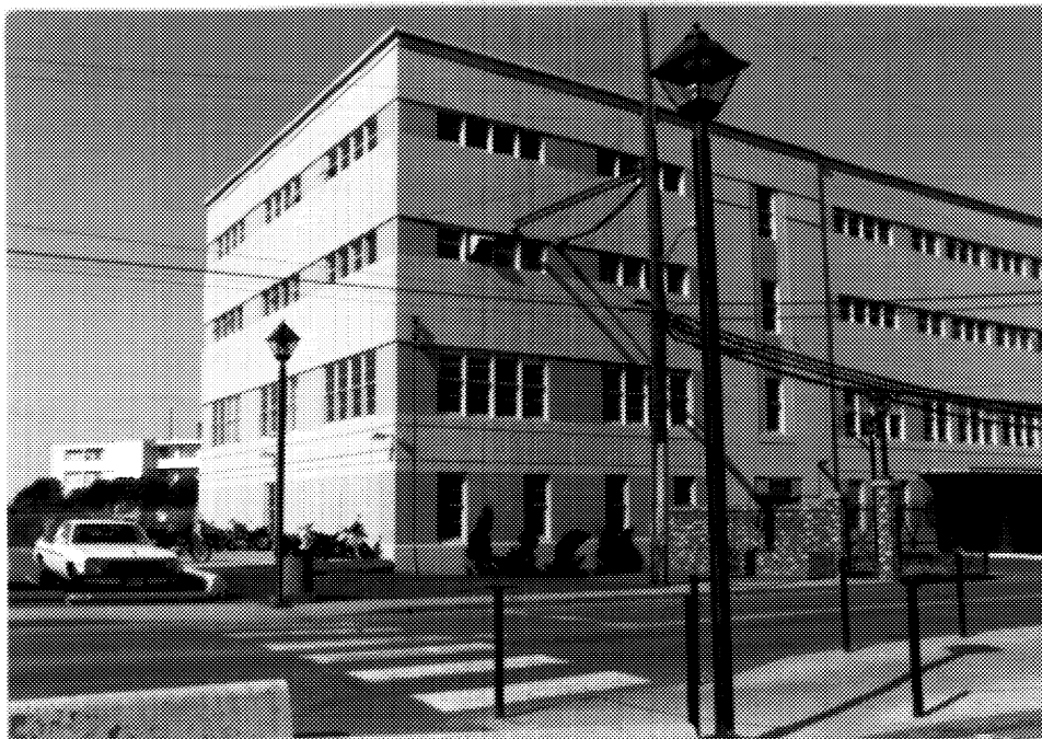
3 Building D211, main and side (east) elevations; building D199 is seen at left, main gate details at left-centre. ( Ian Doull, AHB, Parks, 1989. )
