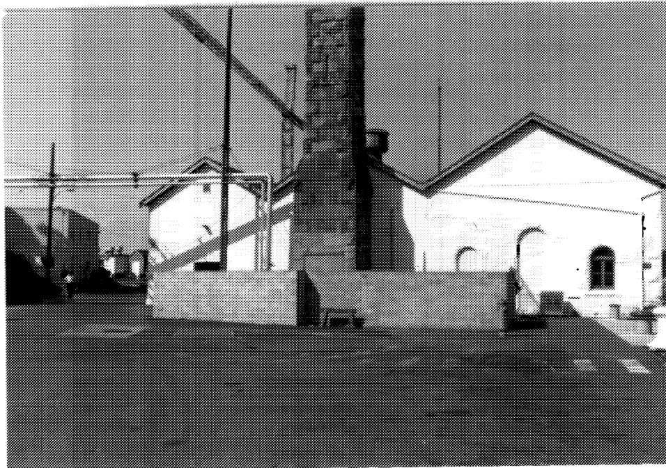
4 Building D175, southern elevation; building D176 stands at left. ( Ian Doull, AHB, Parks, 1989. )
