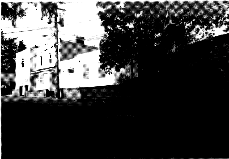
3 Building D25, main elevation. ( Ian Doull, AHB, Parks, 1989. )
