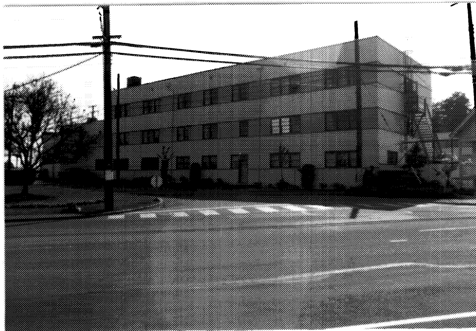
6 Building D11B, eastern elevation. (Ian Doull, AHB, Parks, 1989.)
