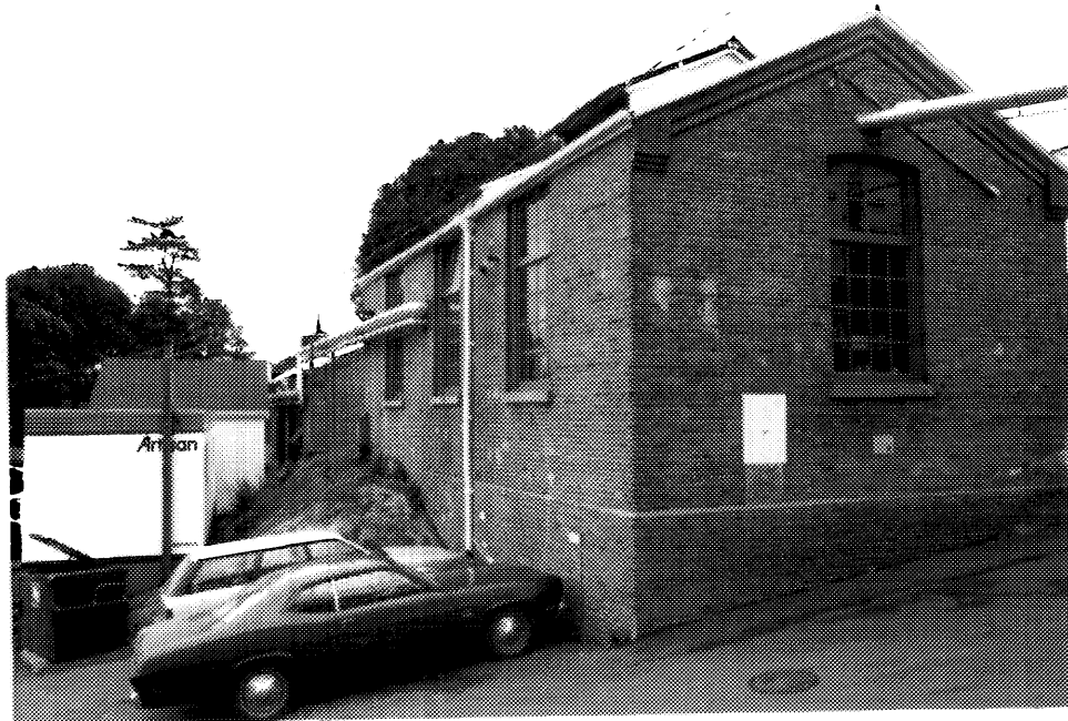
4 Building D59, end (northern) and side (eastern) elevations. Note outcrop, temporary construction trailer to left, buildings D58, D57, mid-left. ( Ian Doull, AHB, Parks, 1989. )
