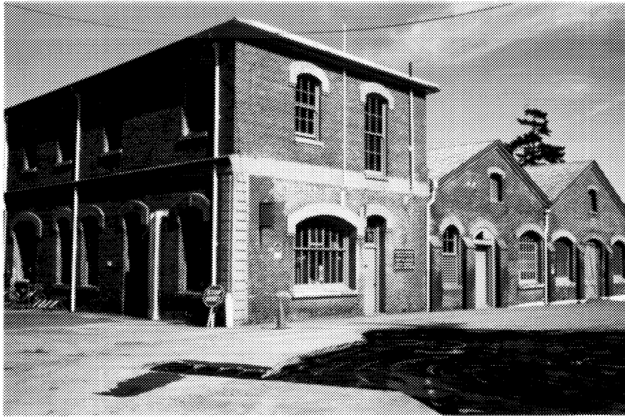
2 Building D51, main (western) and side (northern) elevations. ( Ian Doull, AHB, Parks, 1989. )
