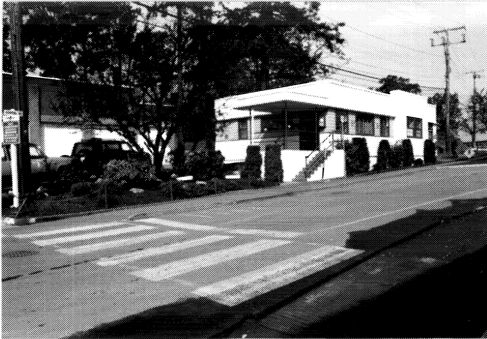
2 Building D37, end (southern) and side (eastern) elevations; building D36 stands at left. (Ian Doull, AHB, Parks, 1989.)
