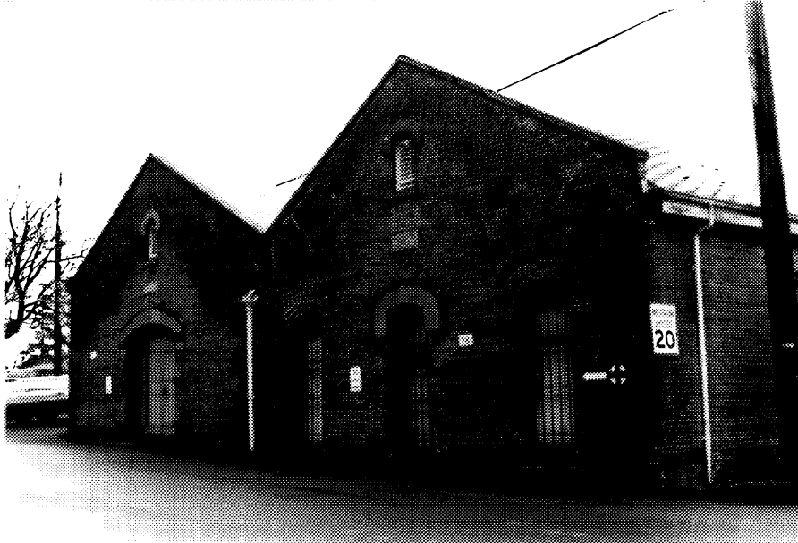
4 Buildings D75-D76. Note changes in door and window openings, performed since 1970. ( CIHB, Parks, 1970. )
