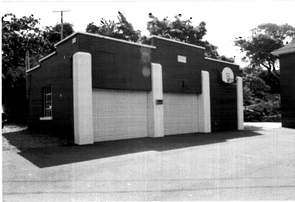
2 Building D102, main (western) and side (northern) elevations. ( Ian Doull, AHB, Parks, 1989. )
