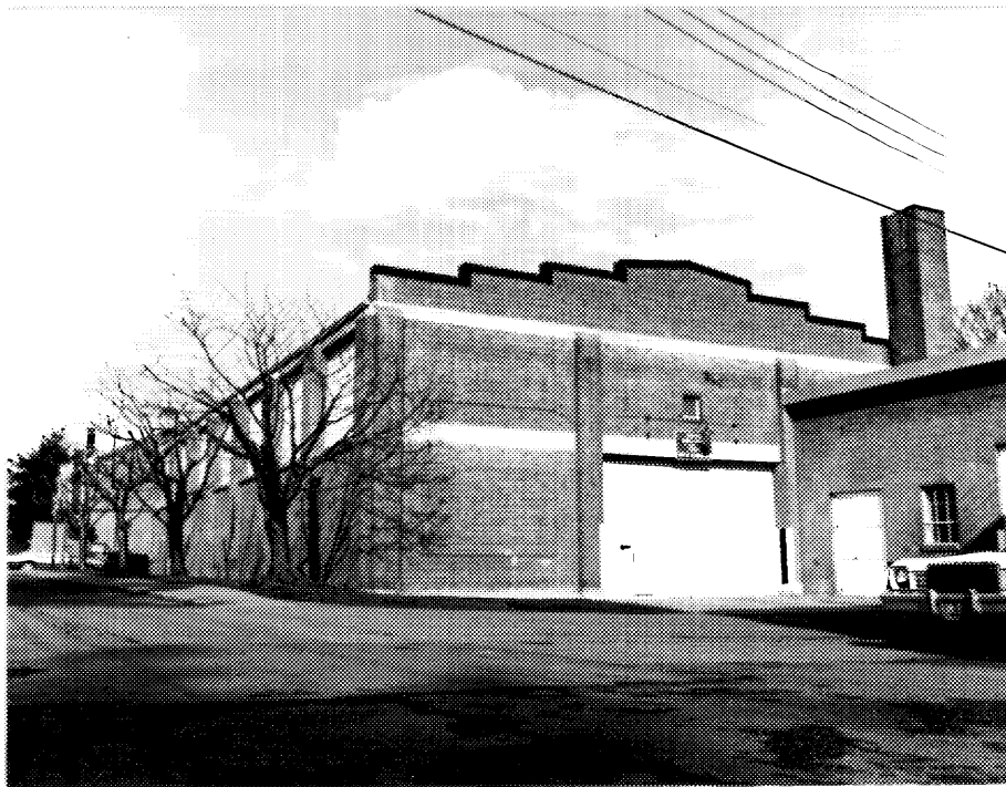
3 Building D22, southern elevation, ca. 1975. ( Canadian forces Photo Unit. )
