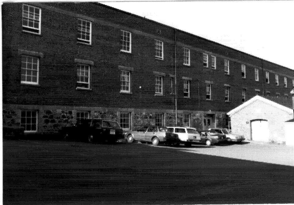
6 Building D109, rear elevation, and building D110. ( Ian Doull, AHB, Parks, 1989. )
