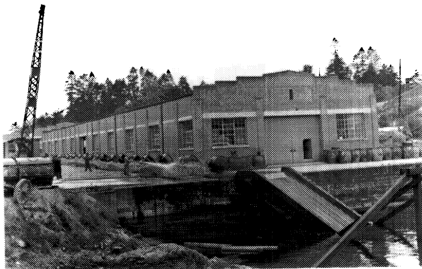
4 Unit D190 and adjacent boom defence net maintenance pad on site of D190A, May 1941. (NA, PA-176365.)
