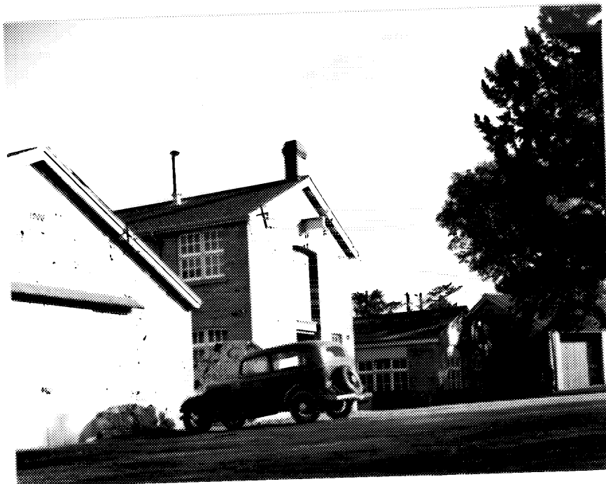
5 Buildings D64, D63, D62, D60, in 1941. (NA, PA-176316. )
