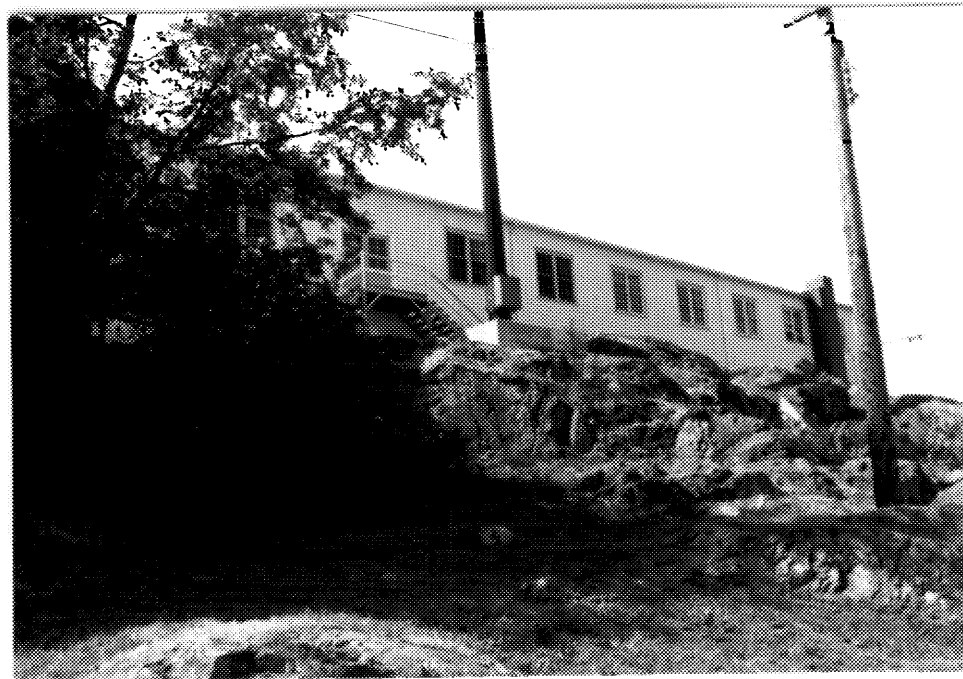
5 Building D178, rear (eastern) elevation, from vicinity of drydock. ( Ian Doull, AHB, Parks, 1989. )
