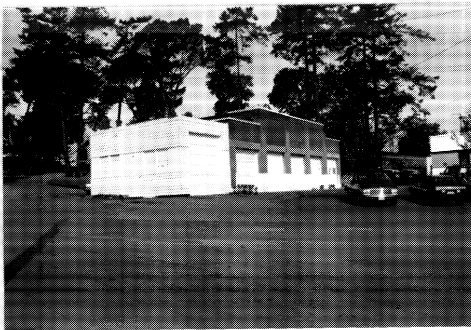
2 Building D36-D36A, main (eastern) and side (southern) elevations. ( Ian Doull, AHB, Parks, 1989. )
