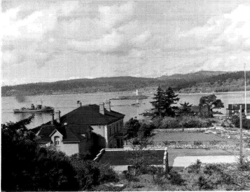
22 Building D101, site details, looking west, 1942. (NA, PA-176340.)
