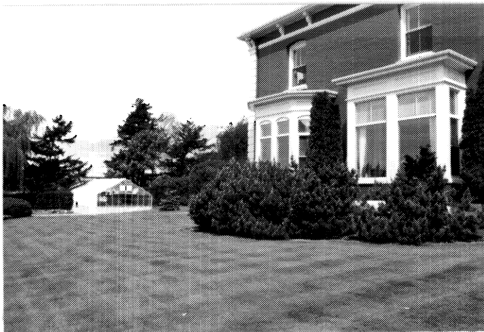
25 Building D101, rear elevation, looking west, and greenhouse. (Ian Doull, AHB, Parks, 1989.)
