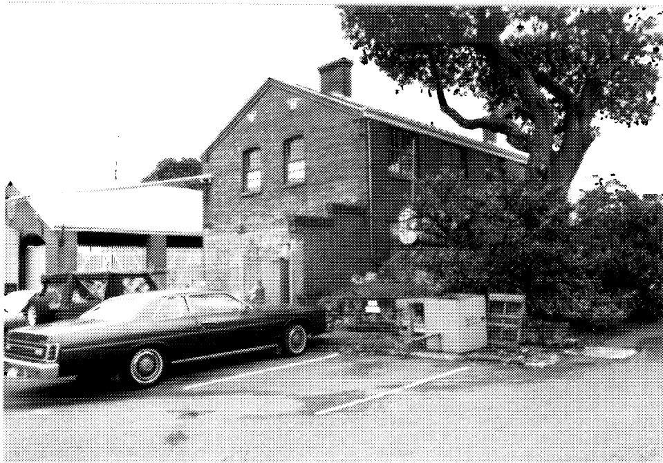
5 Building D68, rear (northern) and side (western) elevations; building D60 stands at left. (Ian Doull, AHB, Parks, 1989.)
