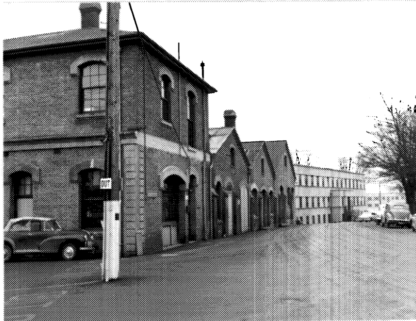
5 Building D51, main elevation, showing demolished southern wing; building D50 at right. (NA, PA-176372.)
