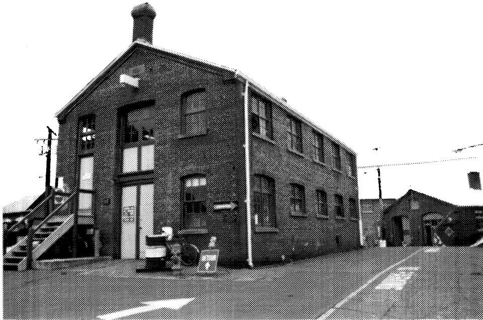
3 Building D68, main (southern) and side (eastern) elevations; building D65 stands at extreme left, buildings D63 and D62 at right. (Ian Doull, AHB, Parks, 1989.)
