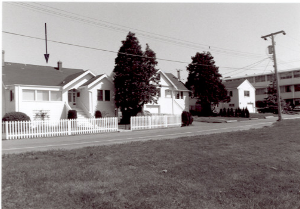
5 Building D195, main (southern) elevation, and D196, D198. ( Ian Doull, AHB, Parks, 1989. )
