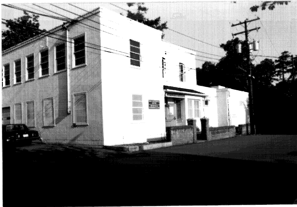
2 Building D25, side (southern) and main (eastern) elevations. ( Ian Doull, AHB, Parks, 1989. )
