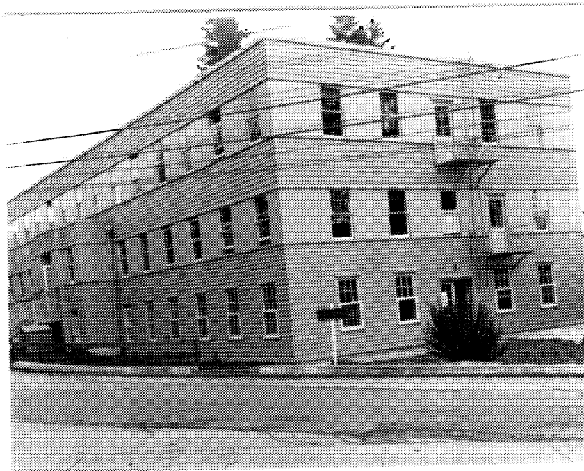
5 Building D50, west and south elevations, October 1942. ( NA, PA-176360. )
