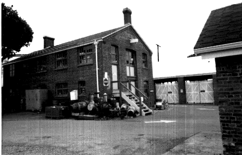
6 Building D68, main and side (western) elevations; buildings D60, D69 stand at right. (Ian Doull, AHB, Parks, 1989.)
