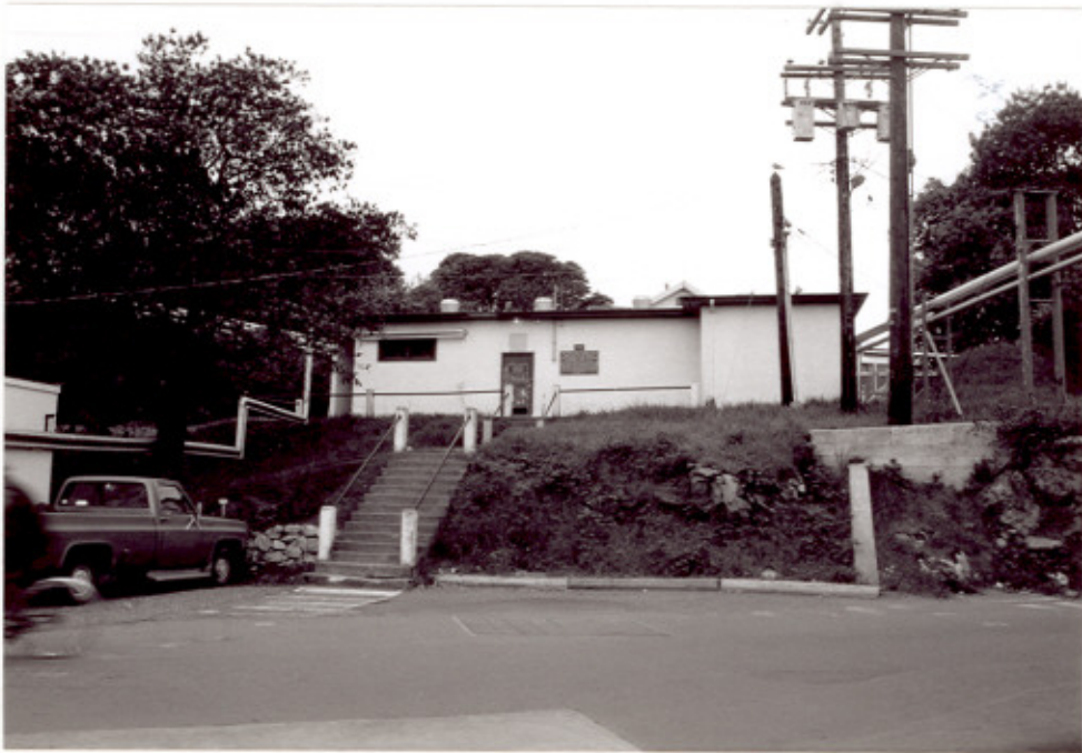
2 Building D172, main (eastern) elevation. ( Ian Doull, AHB, Parks, 1989. )
