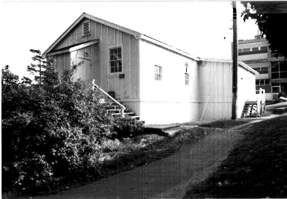
2 Building D223, end (northern) and side (western) elevations; building D218 stands at rear, right. (Ian Doull, AHB, Parks, 1989.)
