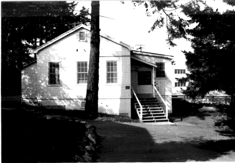
2 Building D217, southern elevation; building D10 stands behind, at right. ( Ian Doull, AHB, Parks, 1989. )
