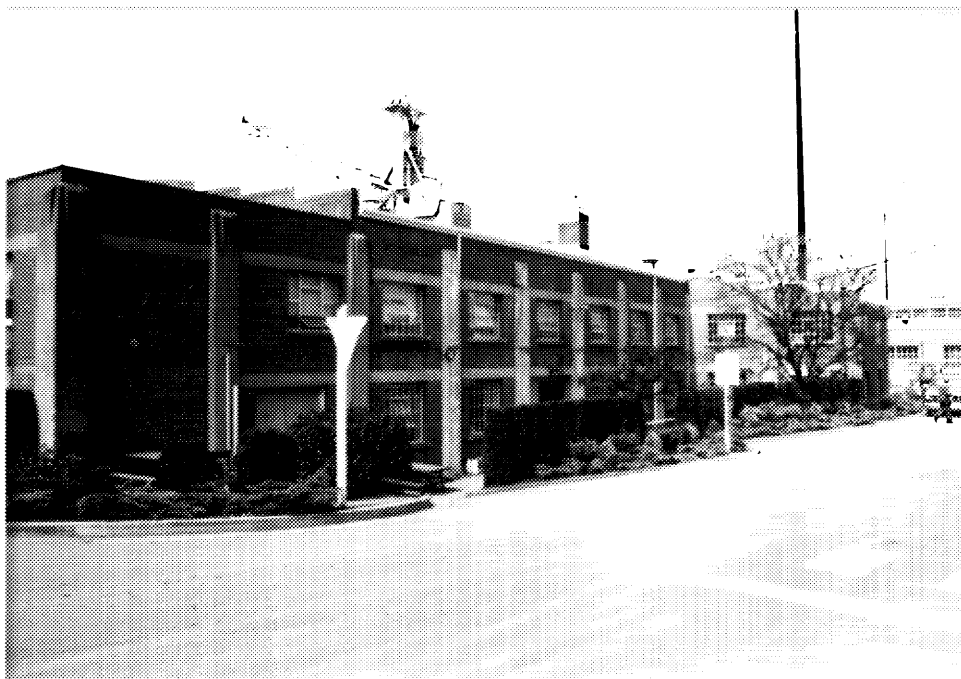
29 Building units D191-D191B, eastern elevation. ( Ian Doull, AHB, Parks, 1989. )
