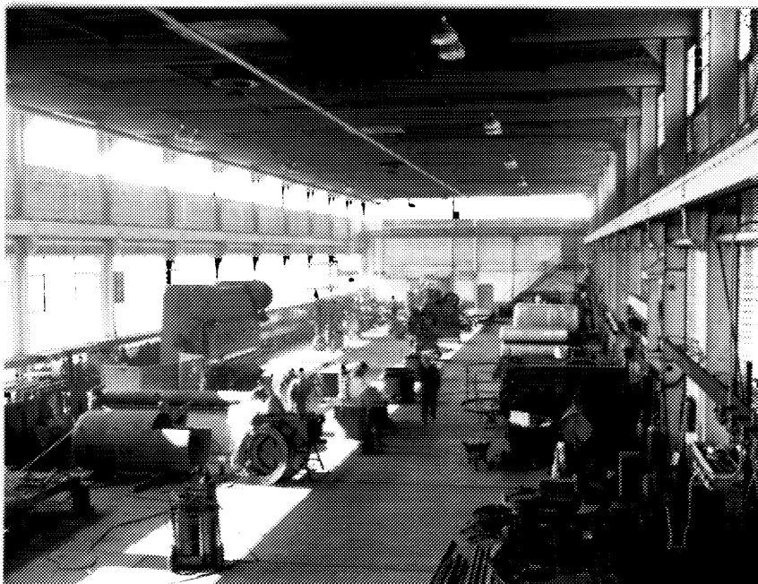
13 Unit D190A, showing interior structural steel framing, 1950. ( NA, PA-176377. )
