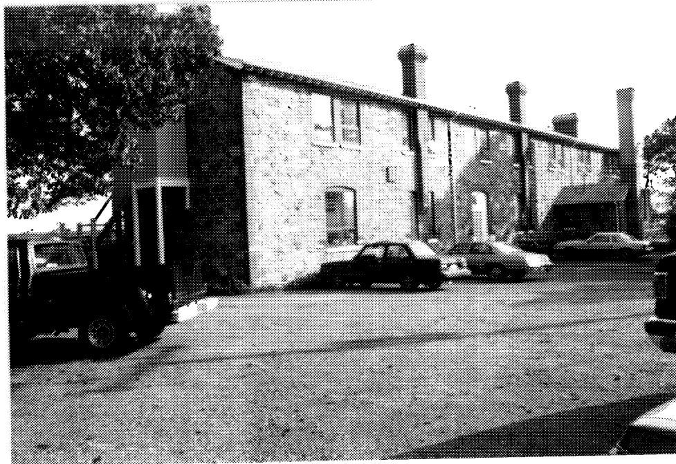
4 Building D38, end (western) and main elevations. (Ian Doull, AHB, Parks, 1989.)
