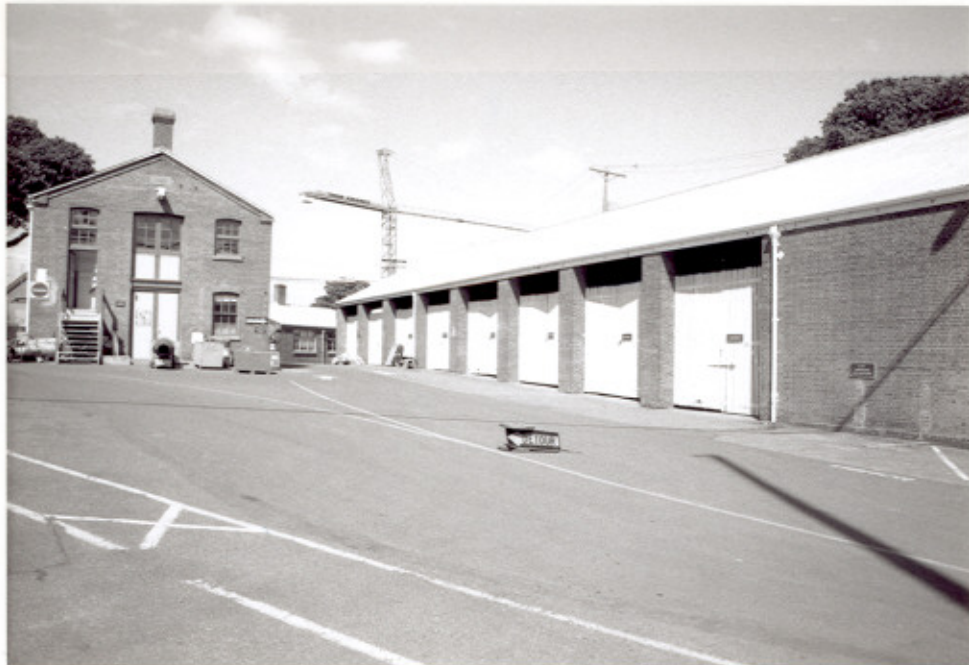
3 Building D60, western elevation; building D68 stands at left. ( Ian Doull, AHB, Parks, 1989. )
