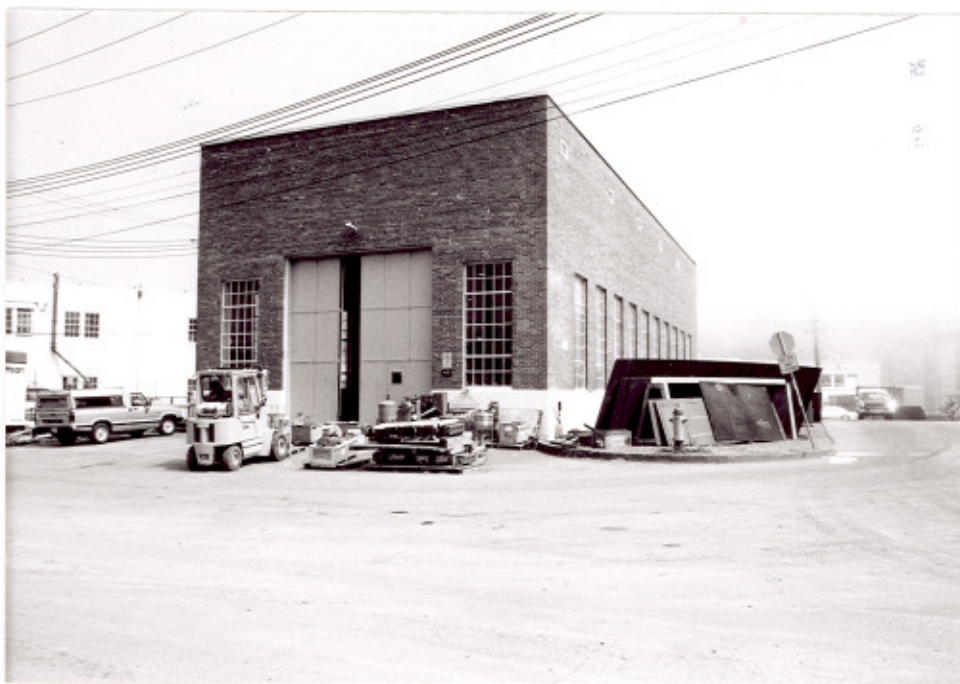
2 Building D142, end (west) and side (south) elevations. (Ian Doull, AHB, Parks, 1989.)
