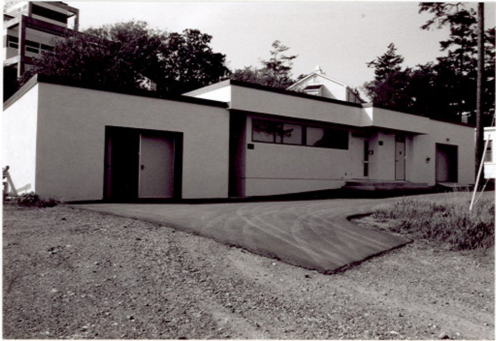
2 Building D9-9A, main (southeastern) elevation; buildings D218, D222, stand above, left and right. (Ian Doull, AHB, Parks, 1989.)
