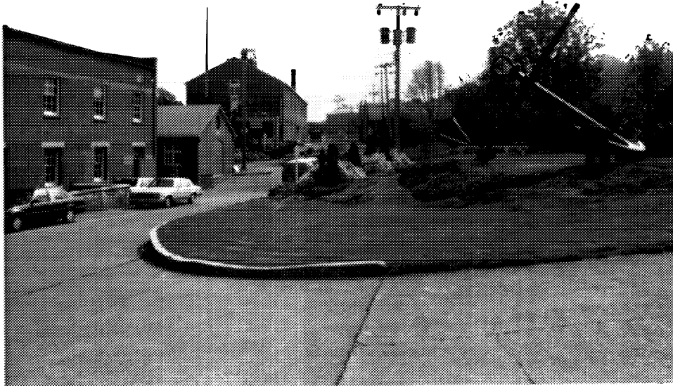
9 Building D109, left, at western end of Hospital Road near Duntze Head. ( Ian Doull, AHB, Parks, 1989. )
