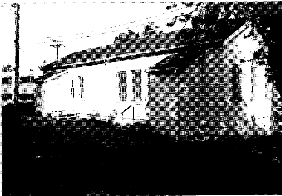
3 Building D217, western elevation; building D10 stands at left. ( Ian Doull, AHB, Parks, 1989. )
