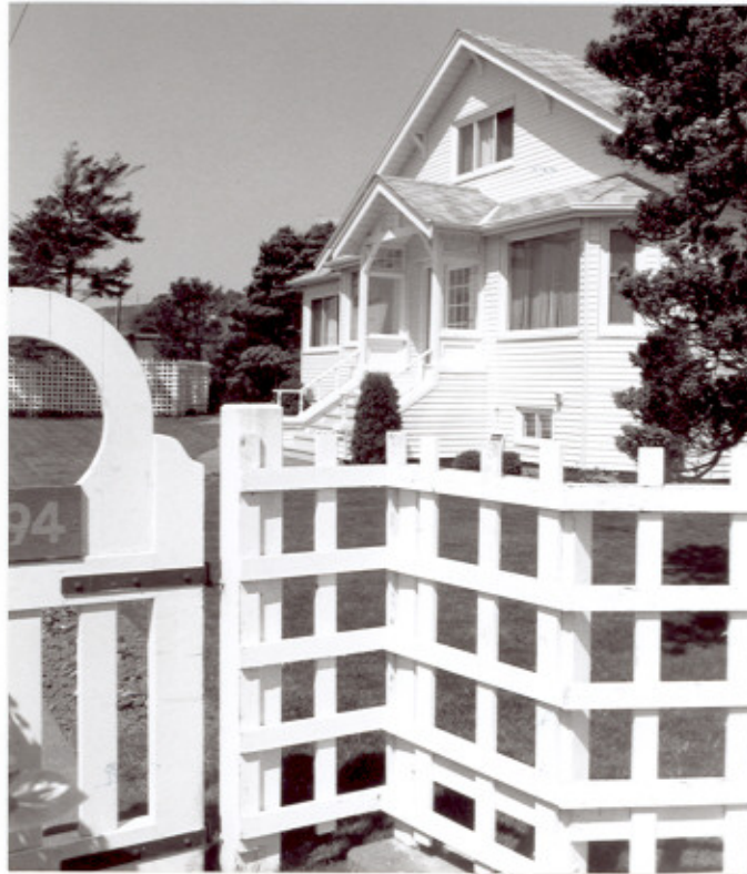
3 Building D194, main elevation. ( Ian Doull, AHB, Parks, 1989. )
