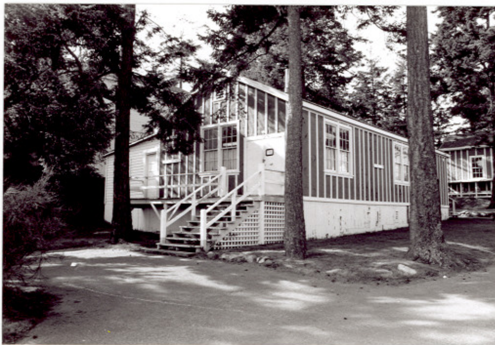
2 Building D244, main (southern) and side (eastern) elevations. ( Ian Doull, AHB, Parks, 1989. )
