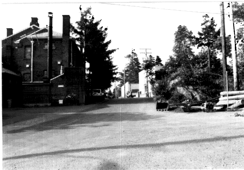
13 Building D26, looking south toward Black Rock; buildings D8, D25 stand at right. ( Ian Doull, AHB, Parks, 1989. )
