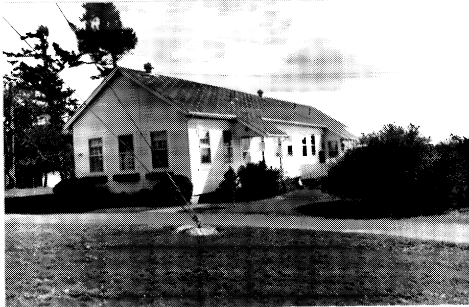
2 Building D106, main (western) and side (northern) elevations, prior to construction of walkway between the entrance porches. ( Canadian Forces Photo Unit. )
