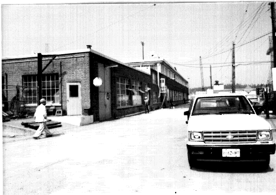
11 Unit 190A, eastern elevation, looking north. ( Ian Doull, AHB, Parks, 1989. )
