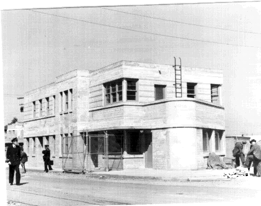
2 Building D214 nearing completion, April 1943, southern and eastern elevations. (NA, PA-176342.)
