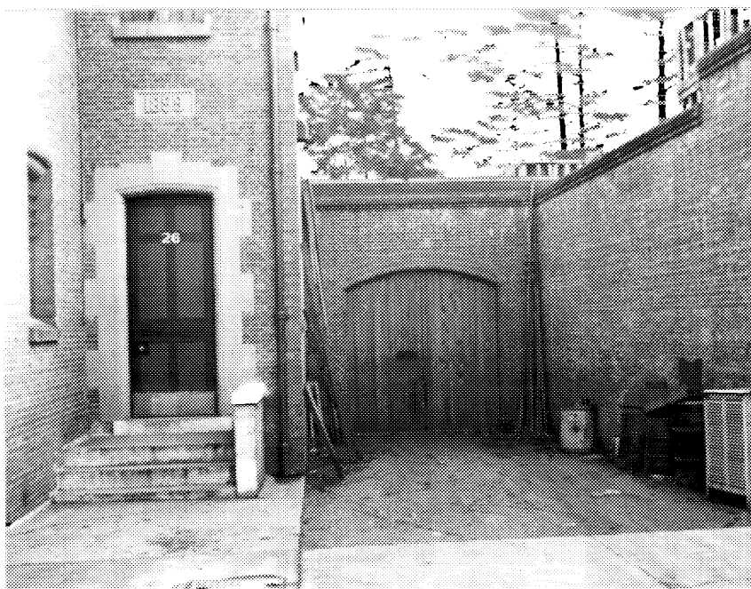
4 Building D26, detail of northwestern door and adjacent wall, 1945. ( NA, PA-176346. )
