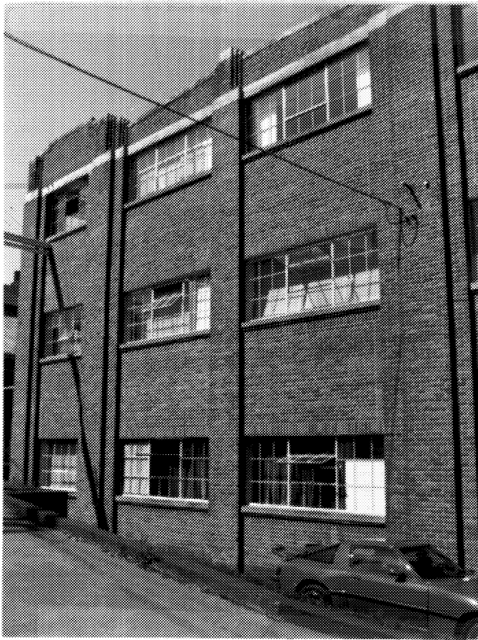
4 Building D83, eastern elevation, detail. (Ian Doull, AHB, Parks, 1989.)
