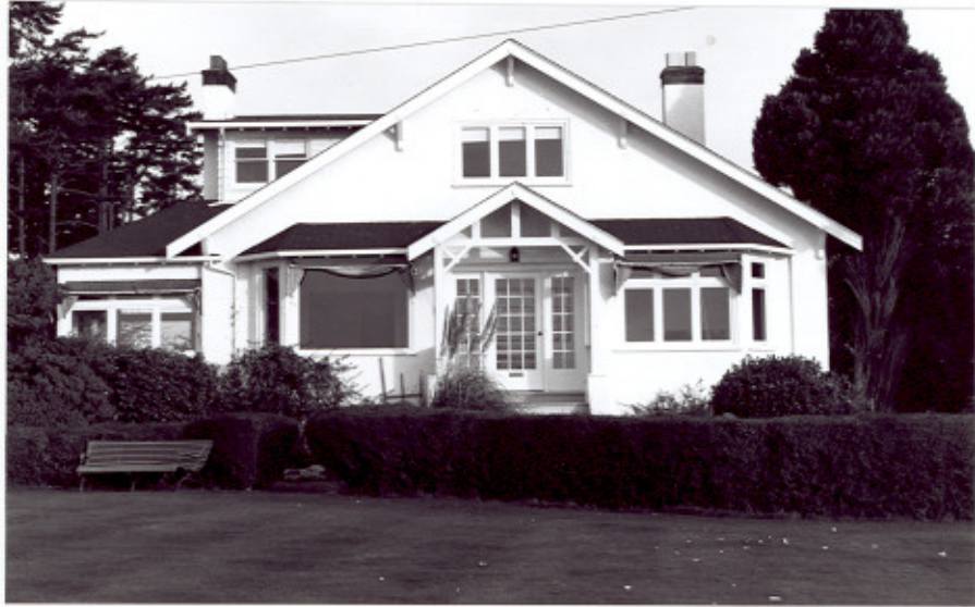
2 Building D194, main (southern) elevation. ( CIHB, Parks, 1976. )
