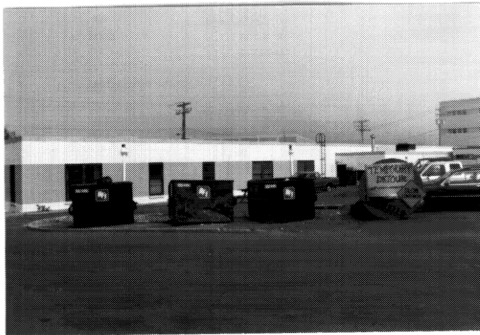
3 Building D210, rear (southern) elevation. ( Ian Doull, AHB, Parks, 1989. )
