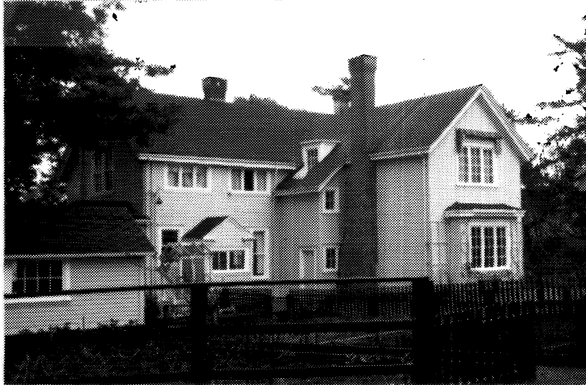
7 Building D1, rear (western) elevations; building D2, base commander's garage, stands at left. ( CIHB, Parks, 1971. )
