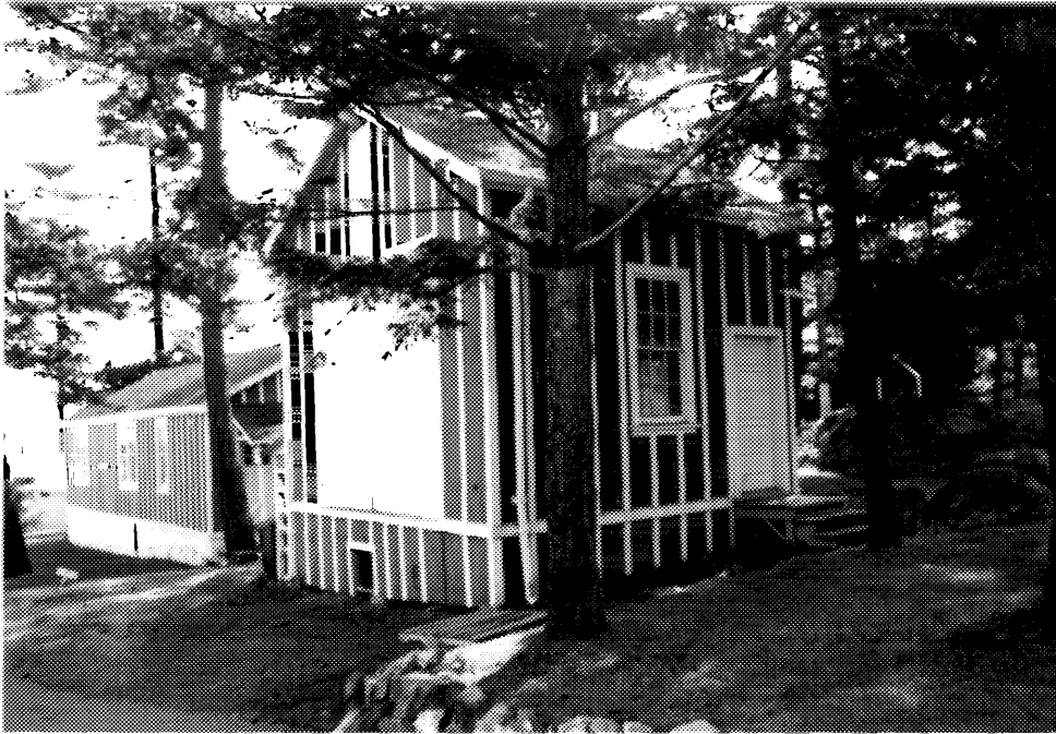
2 Building D224, western and northern sides; building D244 stands at left. ( Ian Doull, AHB, Parks, 1989. )
