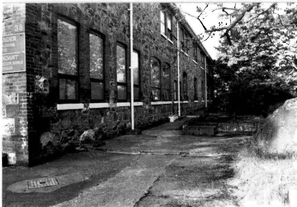
7 Building D38, rear (northern) elevation. ( Ian Doull, AHB, Parks, 1989. )
