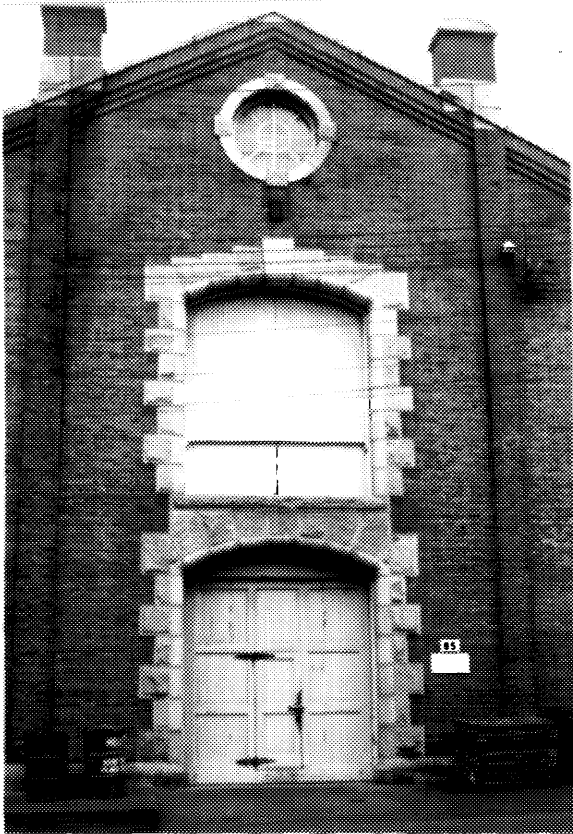
23 Building D85, southern elevation, detail. ( CIHB, Parks, 1974. )
