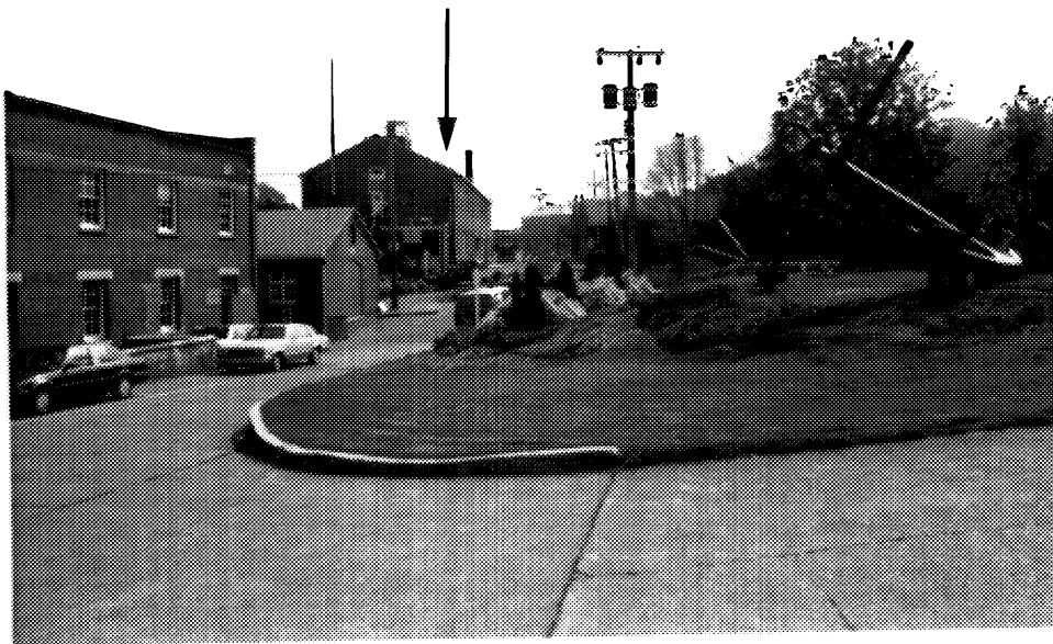
10 Buildings D109, D113, D77 (left to right), from Duntze Head looking east. (Ian Doull, AHB, Parks, 1989.)
