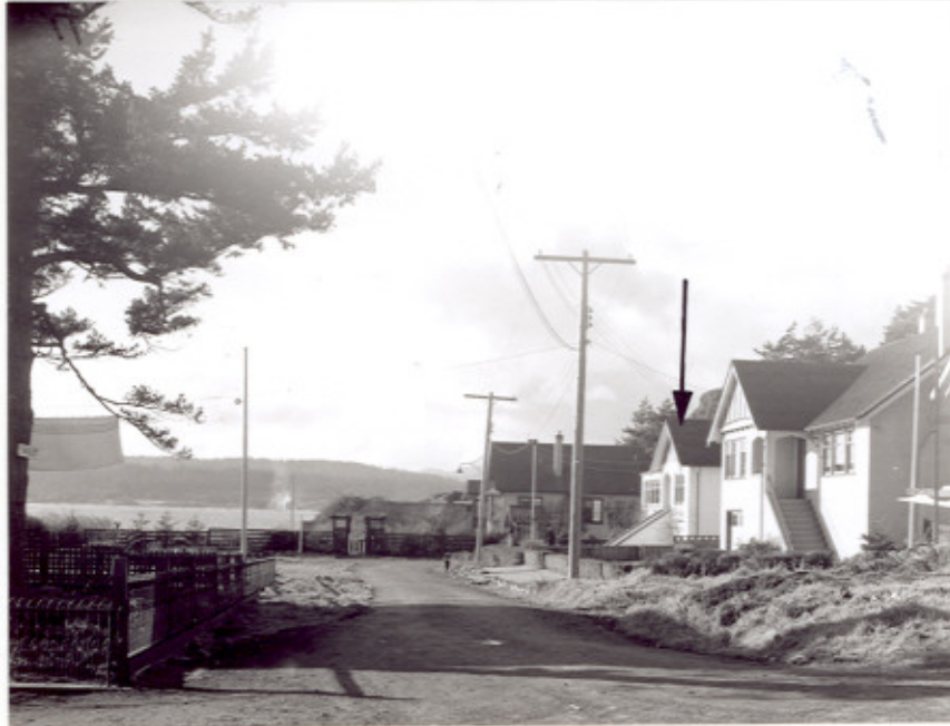
2 Haig Street setting, and buildings D194, D195, D196, January 1942. ( NA, PA-176368. )
