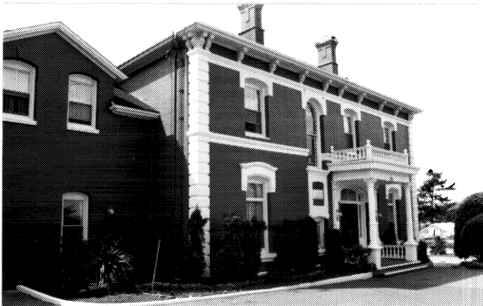
7 Building D101, main elevation. ( Ian Doull, AHB, Parks, 1989. )
