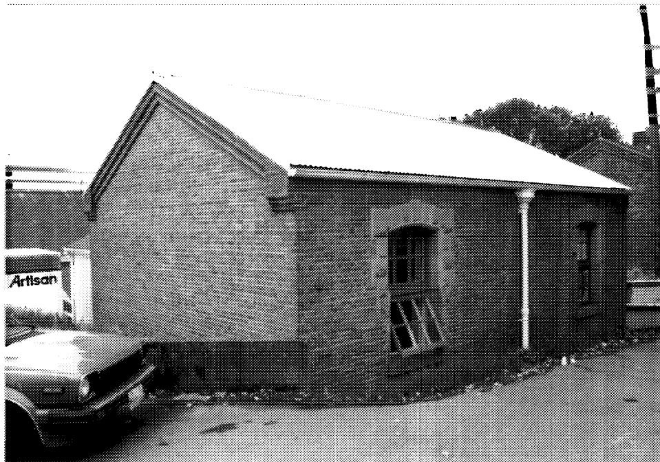
3 Building D57, side and end (northern) elevations. (Ian Doull, AHB, Parks, 1989.)
