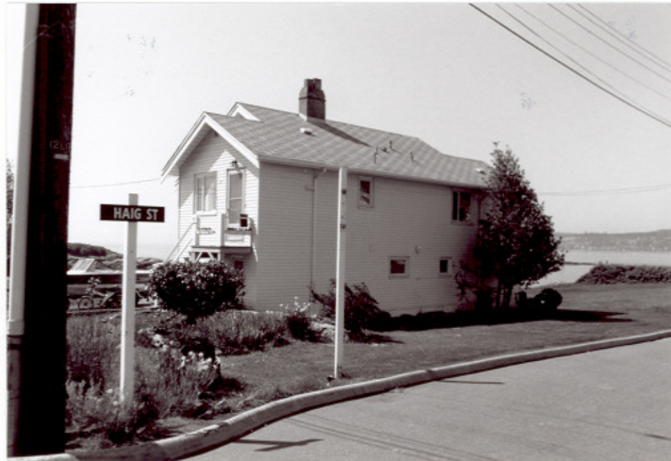
2 Building D197, main (eastern) and side (northern) elevations. ( Ian Doull, AHB, Parks, 1989. )
