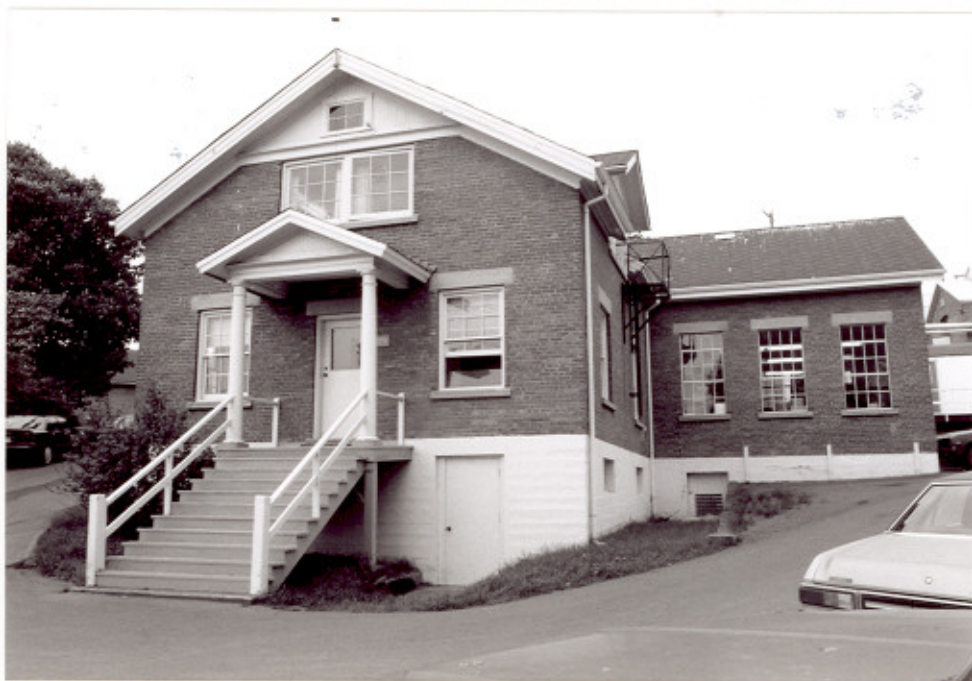
3 Building D179, main (eastern) elevation. ( Ian Doull, AHB, Parks, 1989. )
