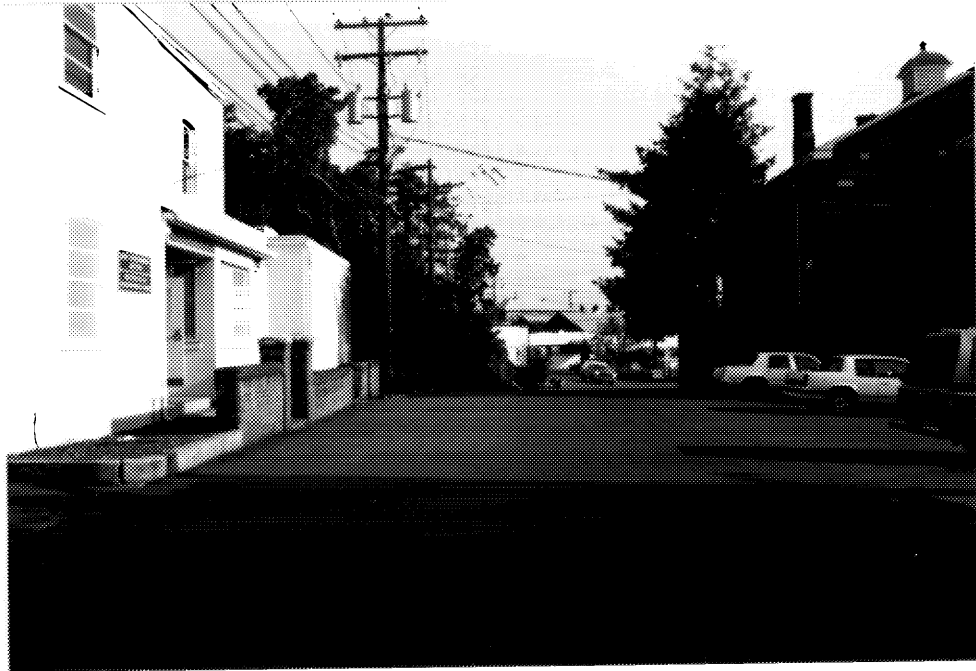
4 Building D25, main elevation, looking north; Hospital Road appears at centre, rear, building D26 stands at right. ( Ian Doull, AHB, Parks, 1989. )
