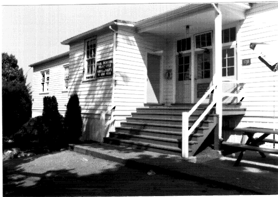
2 Building D178, main (western) elevation, northern end. ( Ian Doull, AHB, Parks, 1989. )
