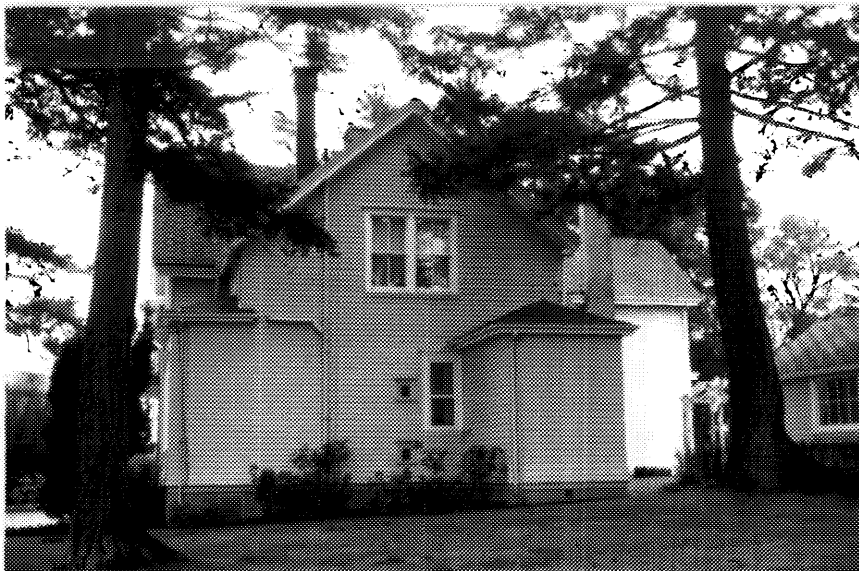
8 Building D1, side (north) elevation. ( CIHB, Parks, 1971. )
