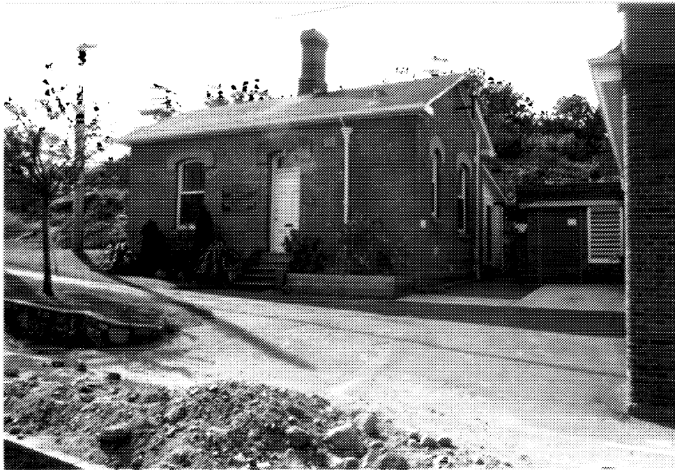
2 Building D74, main (north) and side (east) elevations; building D75 stands at extreme right. ( Ian Doull, AHB, Parks, 1989. )
