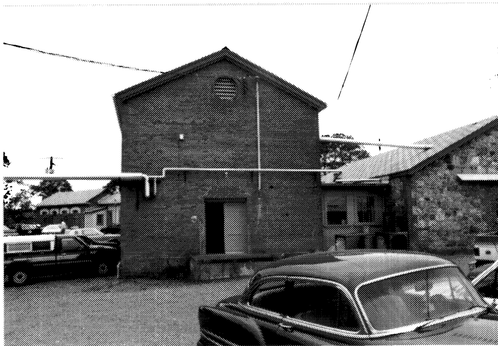
3 Building D63, rear (east) elevation; building D65 stands at left, D64 at right. ( Ian Doull, AHB, Parks, 1989. )
