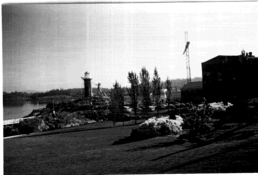
7 Building D109, side (western) elevation, looking north from Duntze Head to Bickford Tower and Grant Knoll. ( Ian Doull, AHB, Parks, 1989. )
