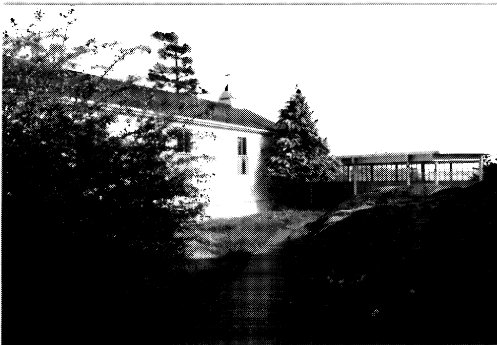
3 Building D222, western elevation and south-end entrance ramp. (Ian Doull, AHB, Parks, 1989.)
