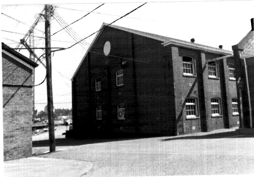
4 Building D80, end and rear (southern) elevations. (Ian Doull, AHB, Parks, 1989.)
