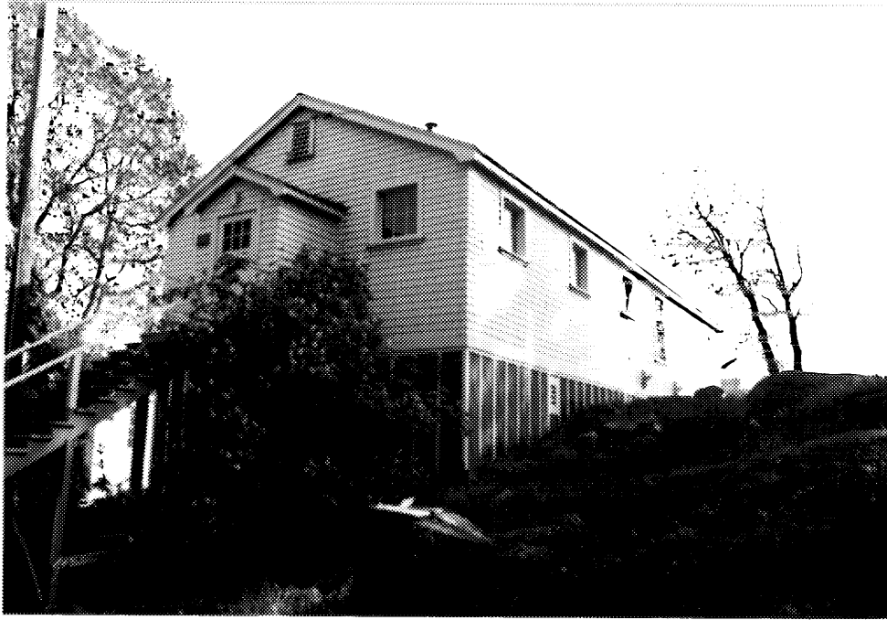
2 Building D219, main (northern) and side (western) elevations. ( Ian Doull, AHB, Parks, 1989. )
