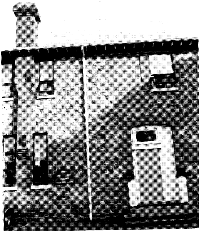
5 Building D38, main elevation, detail. ( Ian Doull, AHB, Parks, 1989. )
