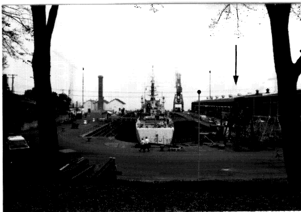
14 "Naden" drydock, with pumphouse (D175) at left, D190-D191 at right. ( Ian Doull, AHB, Parks, 1989. )
