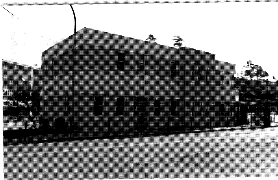
4 Building D214, west and south elevations; building D215 is visible at left. (Ian Doull, AHB, Parks, 1989.)
