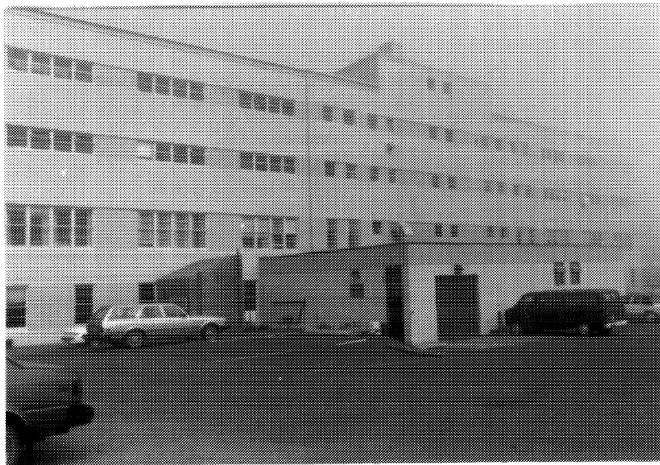
4 Building D211, rear (southern) elevation. ( Ian Doull, AHB, Parks, 1989. )
