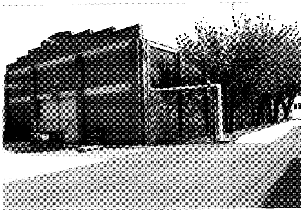
5 Building D22, end (northern) and side (western) elevations. ( Ian Doull, AHB, Parks, 1989. )
