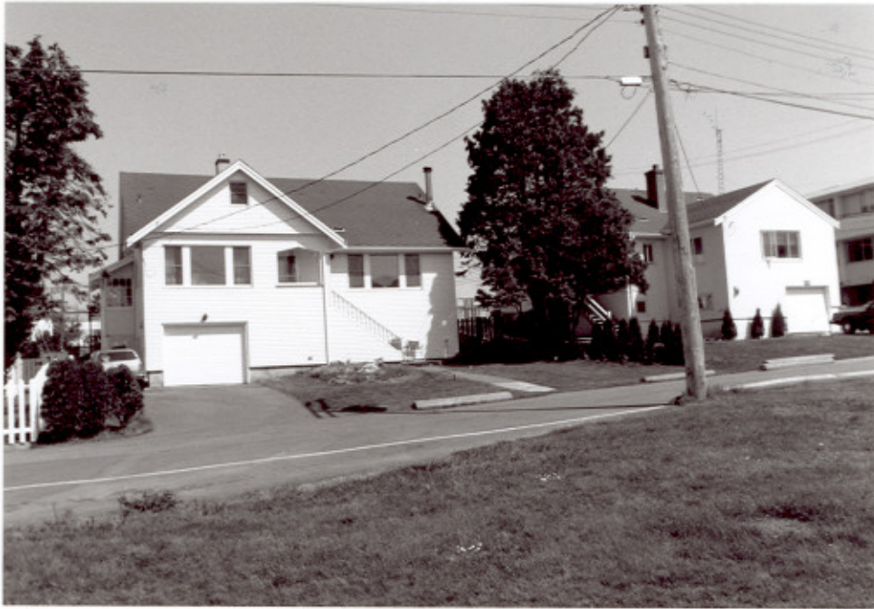
2 Building D196, main (southern) elevation; building D198 stands at right. ( Ian Doull, AHB, Parks, 1989. )
