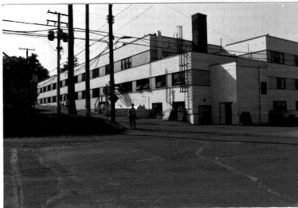
7 Building D11A, rear elevation. ( Ian Doull , AHB, Parks, 1989. )
