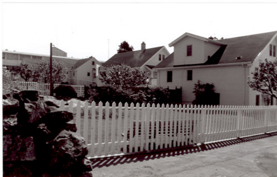
7 Building D195, rear (northern) elevation and landscape; D196, D198 stand at left. ( Ian Doull, AHB, Parks, 1989. )
