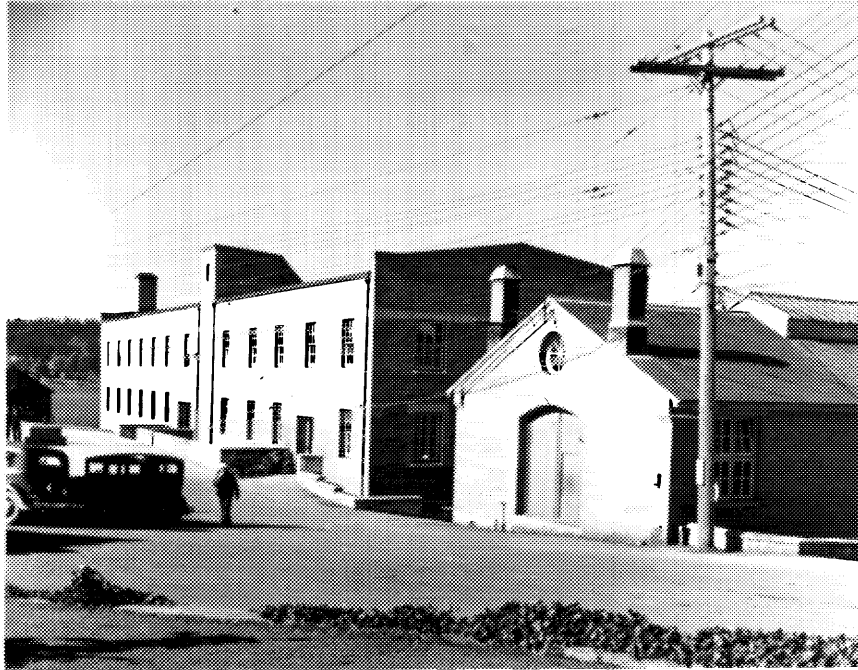
10 Building D113, 1941, showing original chimneys and roof detail; building D109 appears at left. (NA, PA-176318.)
