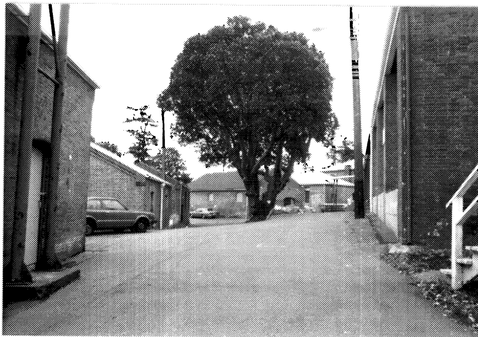
6 "Historic courtyard." Left to right: buildings D59, D57, D55, D51, D60. ( Ian Doull, AHB, Parks, 1989. )
