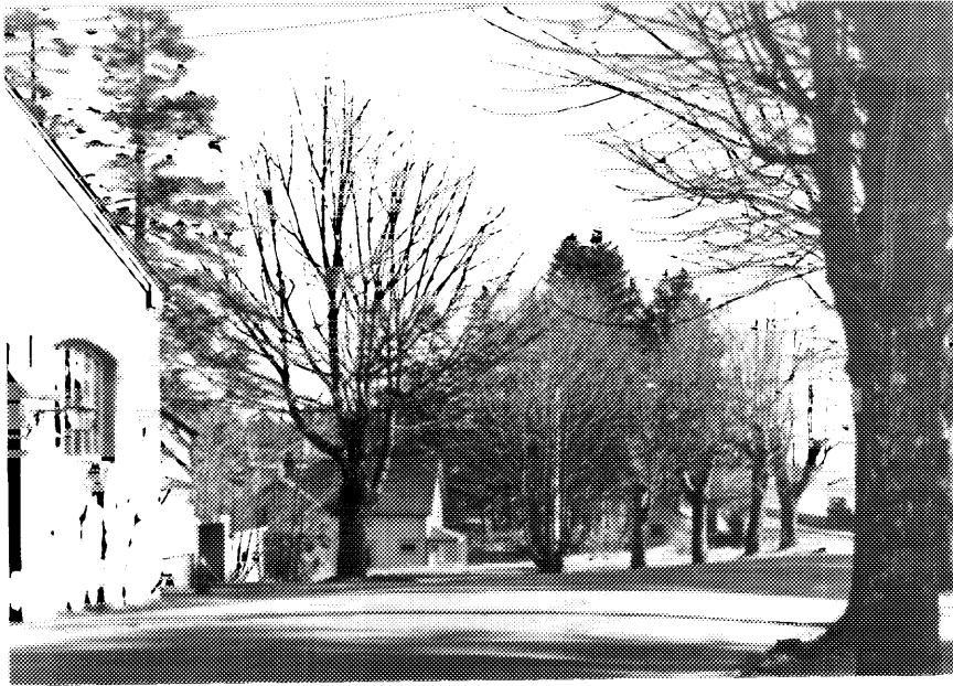
15 Hospital Road, looking southeast from building D51, following removal of original Dockyard gate, February 1941. (NA, PA-176313.)
