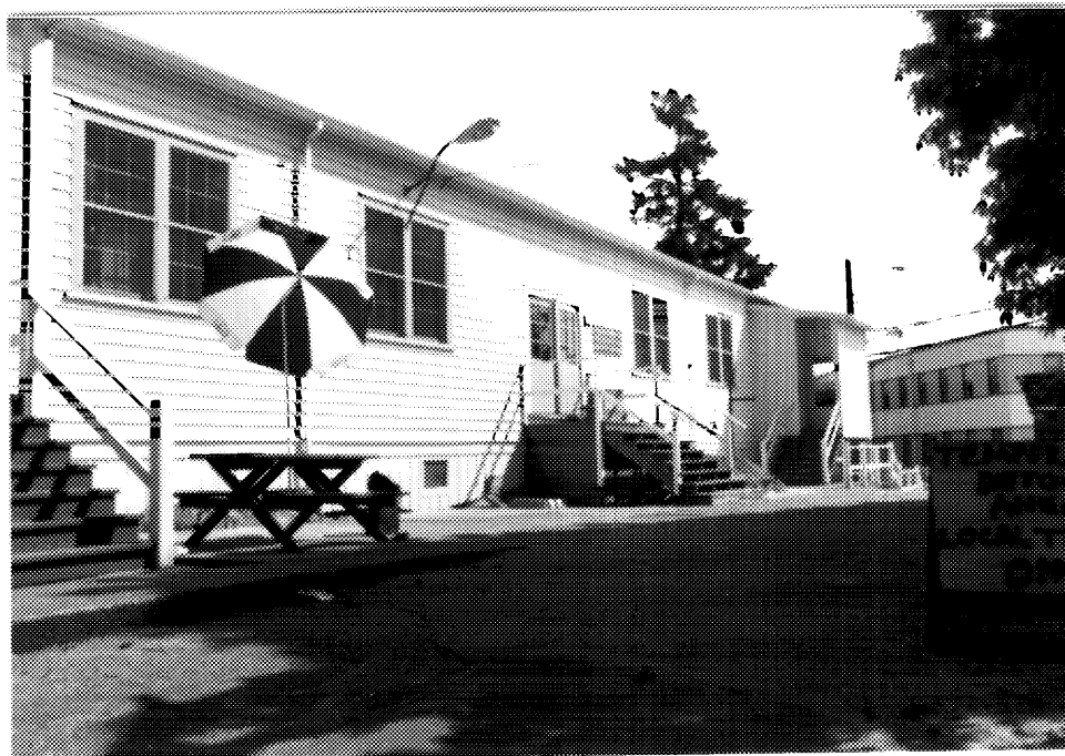
4 Building D178, main elevation, looking south to building D50. ( Ian Doull, AHB, Parks, 1989. )
