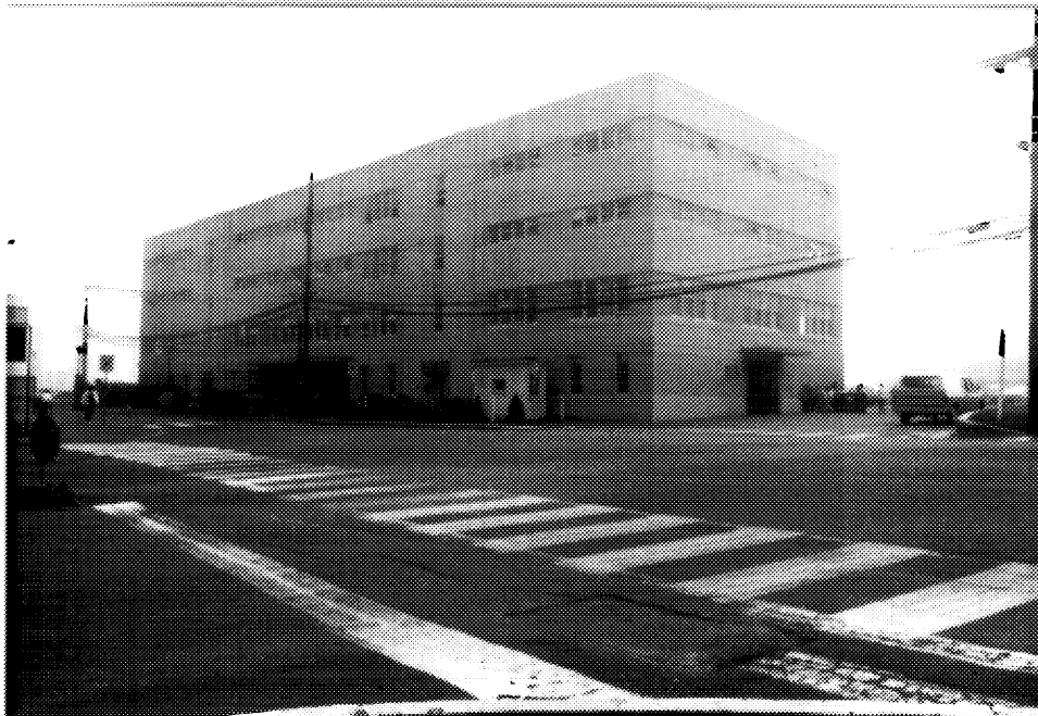
2 Building D211, main (northern) and side (western) elevations. ( Ian Doull, AHB, Parks, 1989. )
