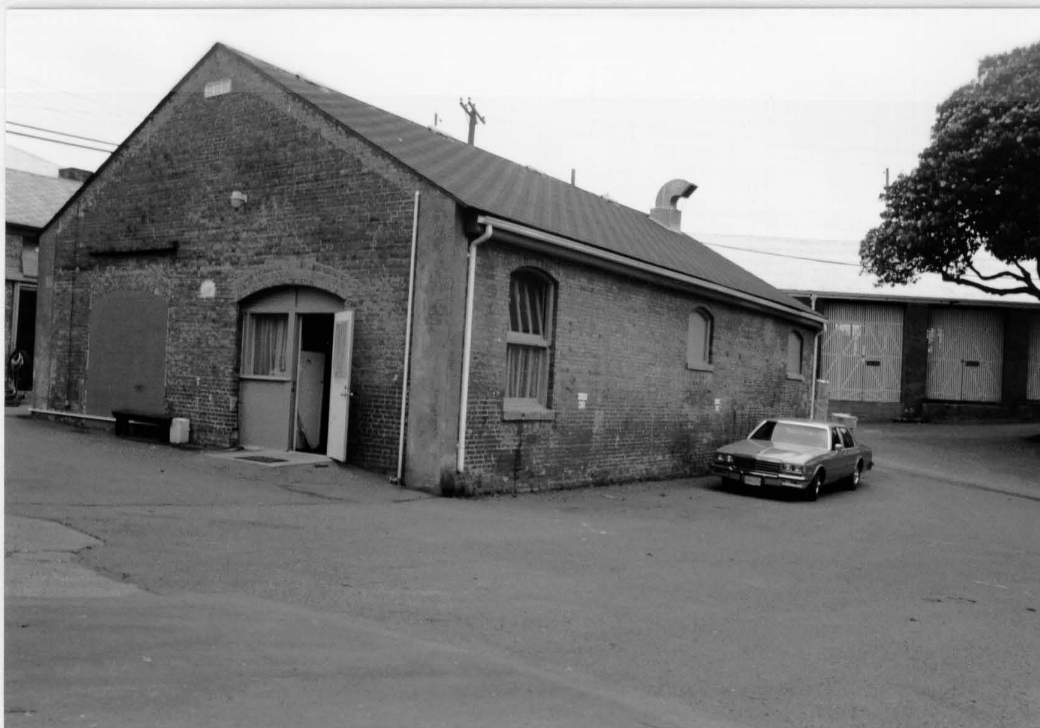
2 Building D55, end (south) and side (east) elevations; building D60 stands at right. ( Ian Doull, AHB, Parks, 1989. )
