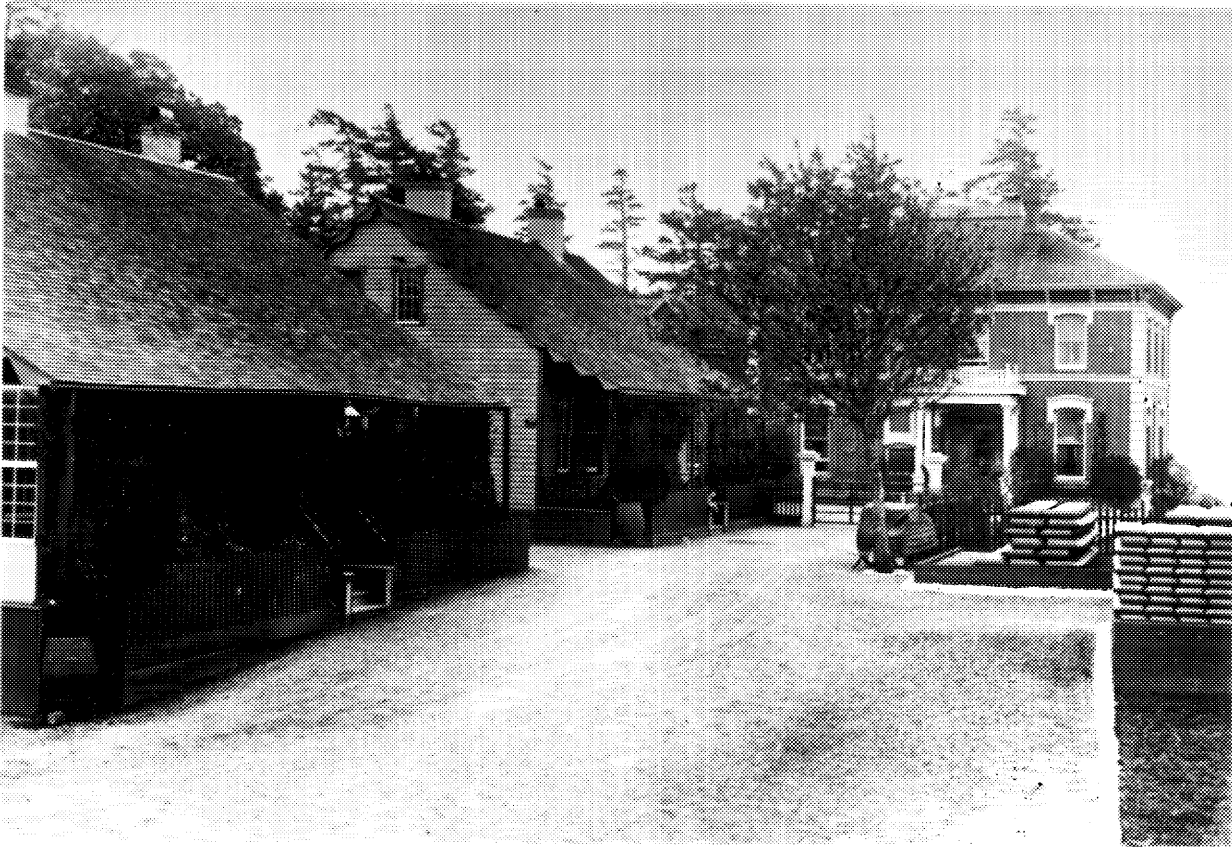
6 Building D101, on site of one of the three original Crimean huts, the surviving examples of which stand at left, ca. 1890. ( NA, C-134131. )
