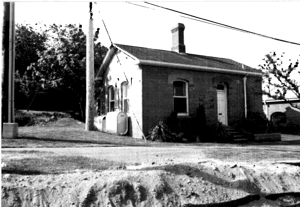
3 Building D74, main and side (west) elevations. ( Ian Doull, AHB, Parks, 1989. )
