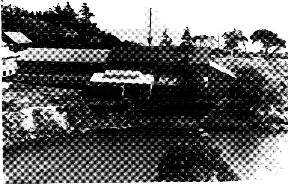
2 Building D109, rear (northern) elevation, with buildings D113, Crimean hut, Admiral's House (D101) at left, D110 at front, centre, 1913. ( Canadian Forces Photo Unit. )
