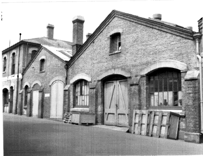
26 Building D51, main (southern) elevation, 1953. ( NA, PA-176353. )
