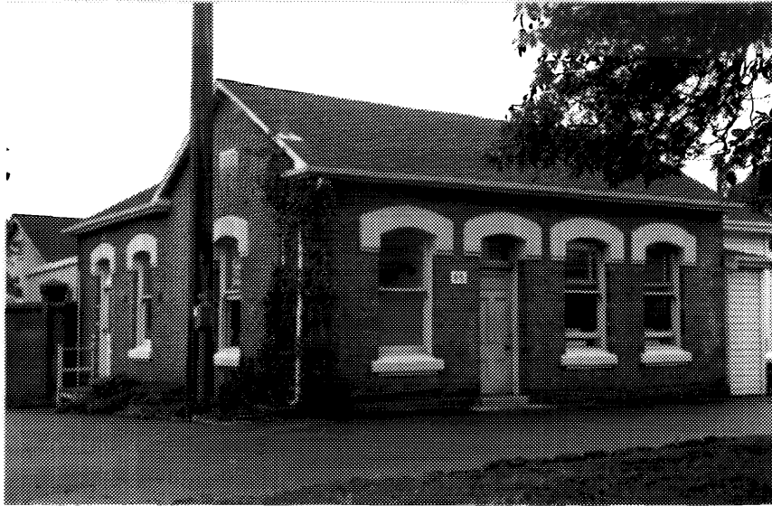
2 Building D65, main (eastern) and side (southern) elevations. ( CIHB, Parks, 1970. )
