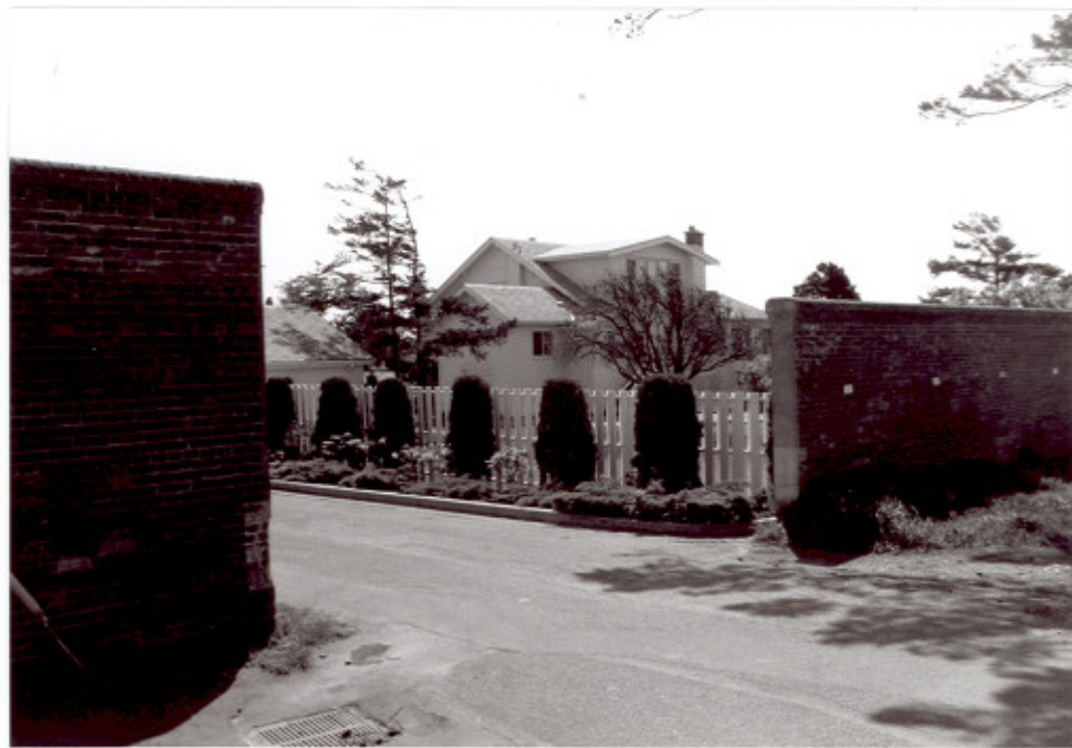
7 Building D194, eastern elevation, viewed through opening in Dockyard wall. (Ian Doull, AHB, Parks, 1989.)
