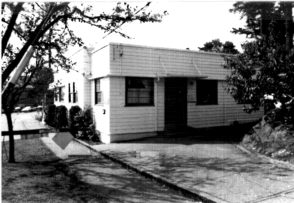
3 Building D37, end (northern) and side elevations. (Ian Doull, AHB, Parks, 1989.)
