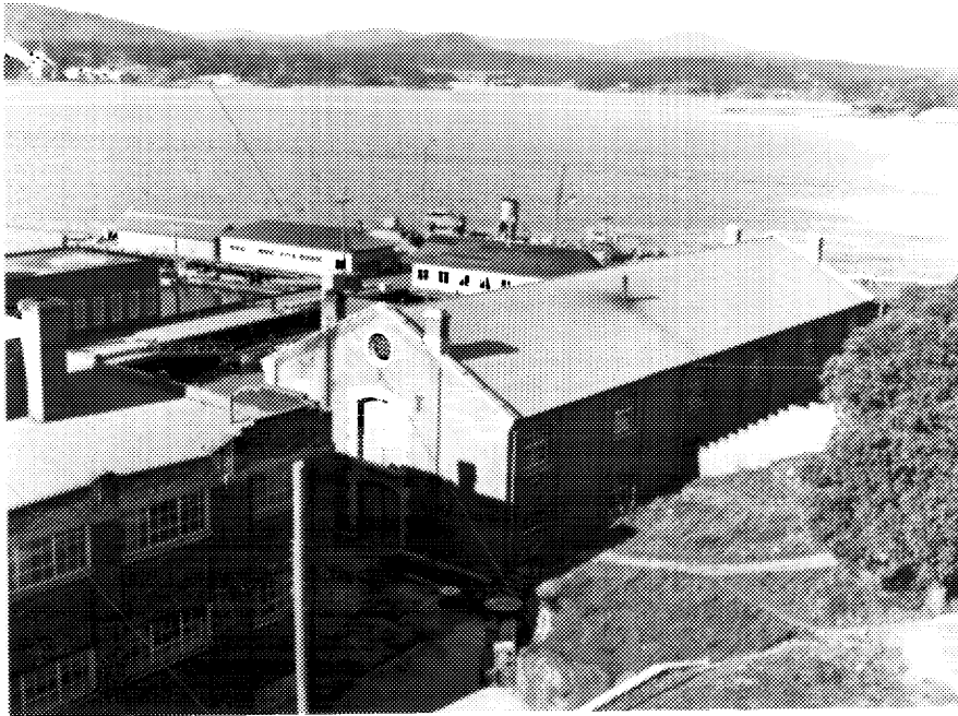
21 Building D85, end (southern) and side (eastern) elevations, 1941. ( NA, PA-176321. )
