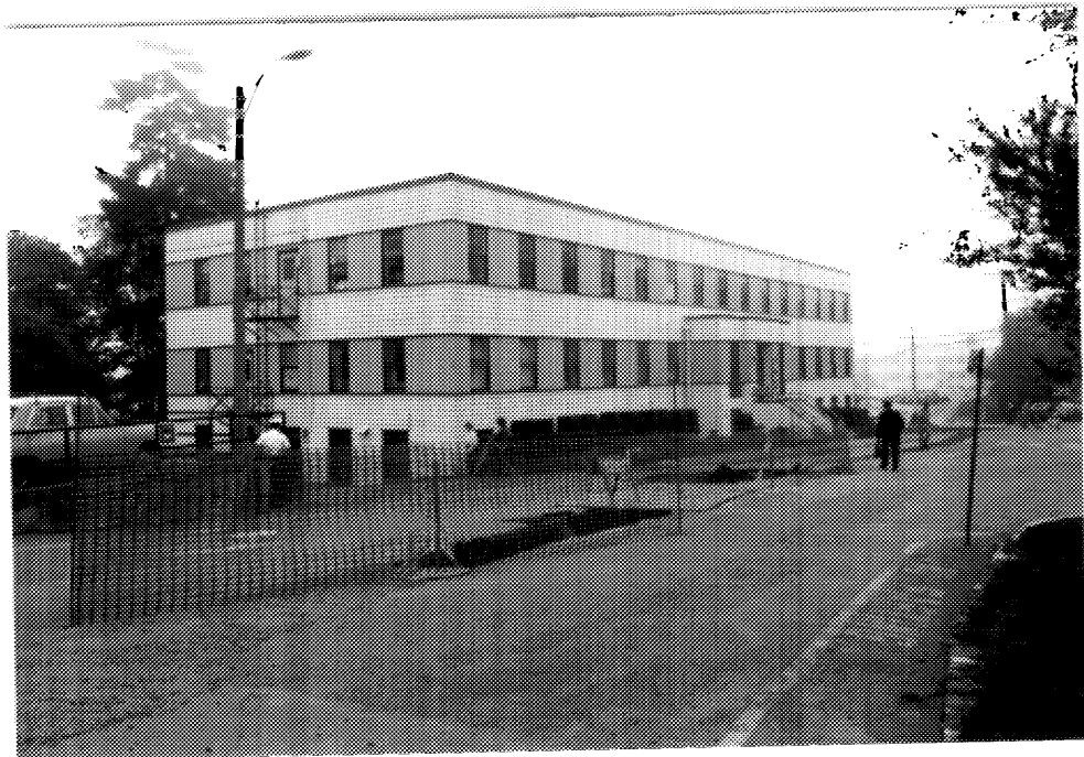
3 Building D50, main and side (north) elevations. ( Ian Doull, AHB, Parks, 1989. )
