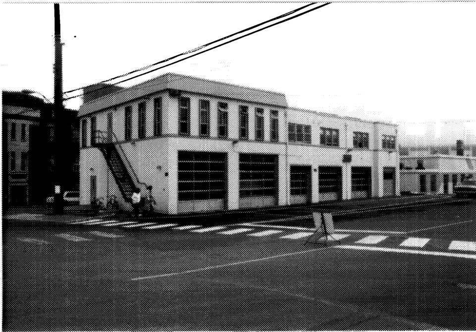
2 Building D212, main (south) and side (west) elevations, showing buildings D192 behind at left; D213 at right. ( Ian Doull, AHB, Parks, 1989. )
