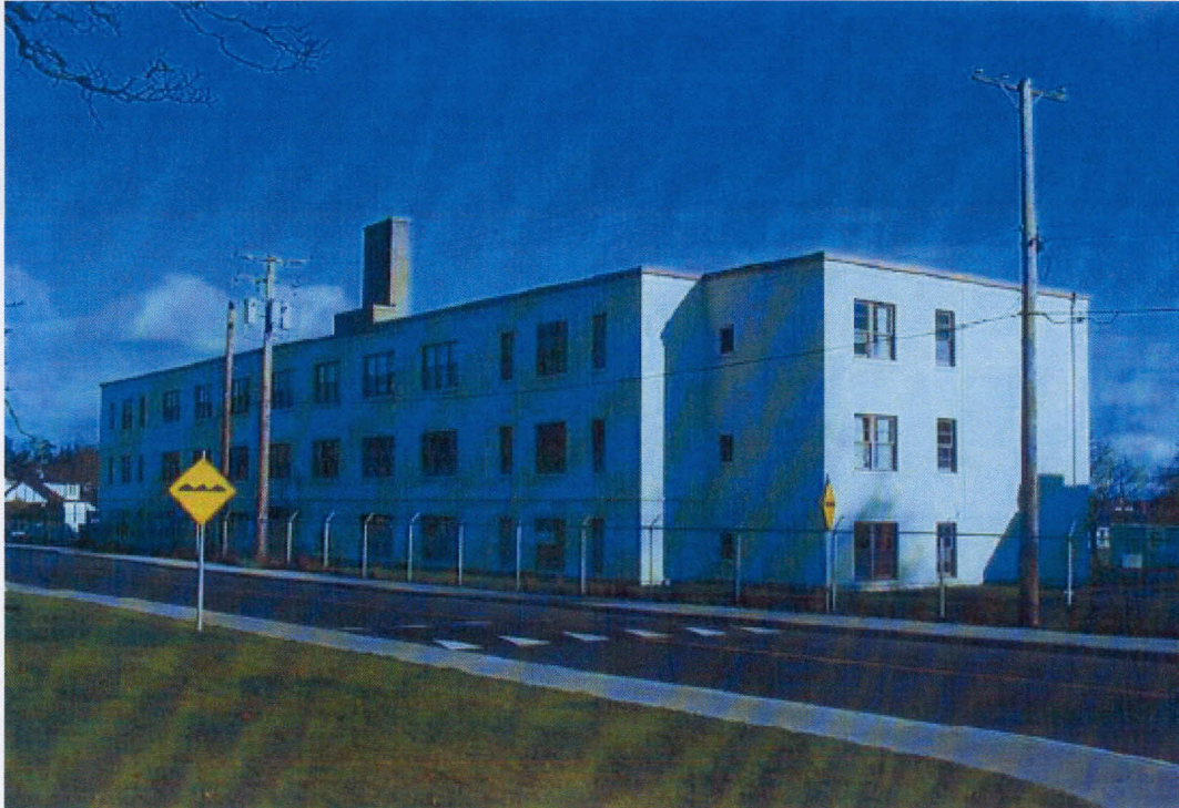
Figure 14. Rear elevation, WP1091, Work Point, CFB Esquimalt (DND, 2011).
