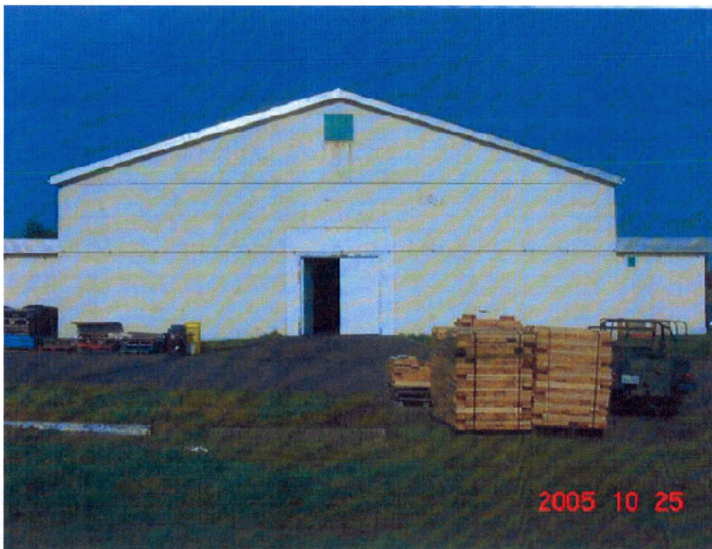
Figure 20. Rear elevation, WP1125, Work Point Barracks, CFB Esquimalt (DND, 2005).
