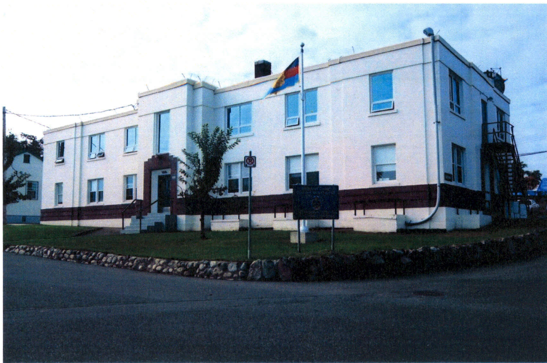
Figure 7. Front elevation, WP1058, Work Point Barracks, CFB Esquimalt (Ian Doull, Parks Canada, 2011).
