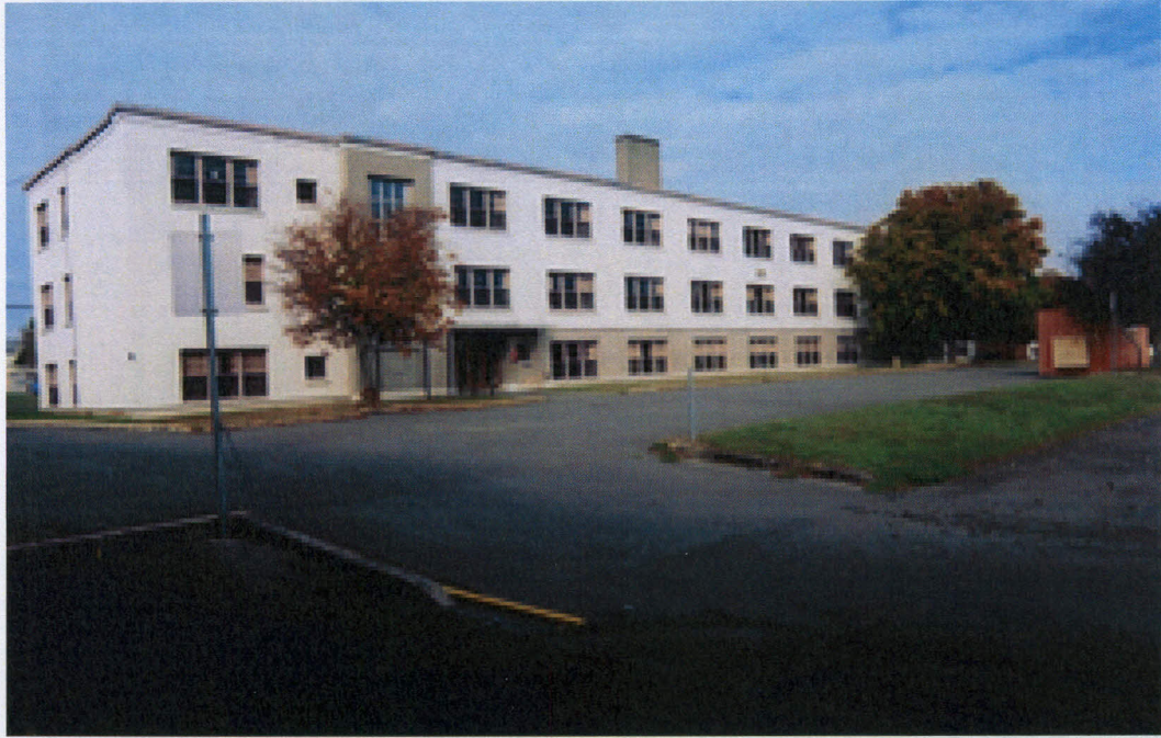
Figure 12. Front elevation, WP1091, Work Point, CFB Esquimalt (Ian Doull, Parks Canada, 2011).
