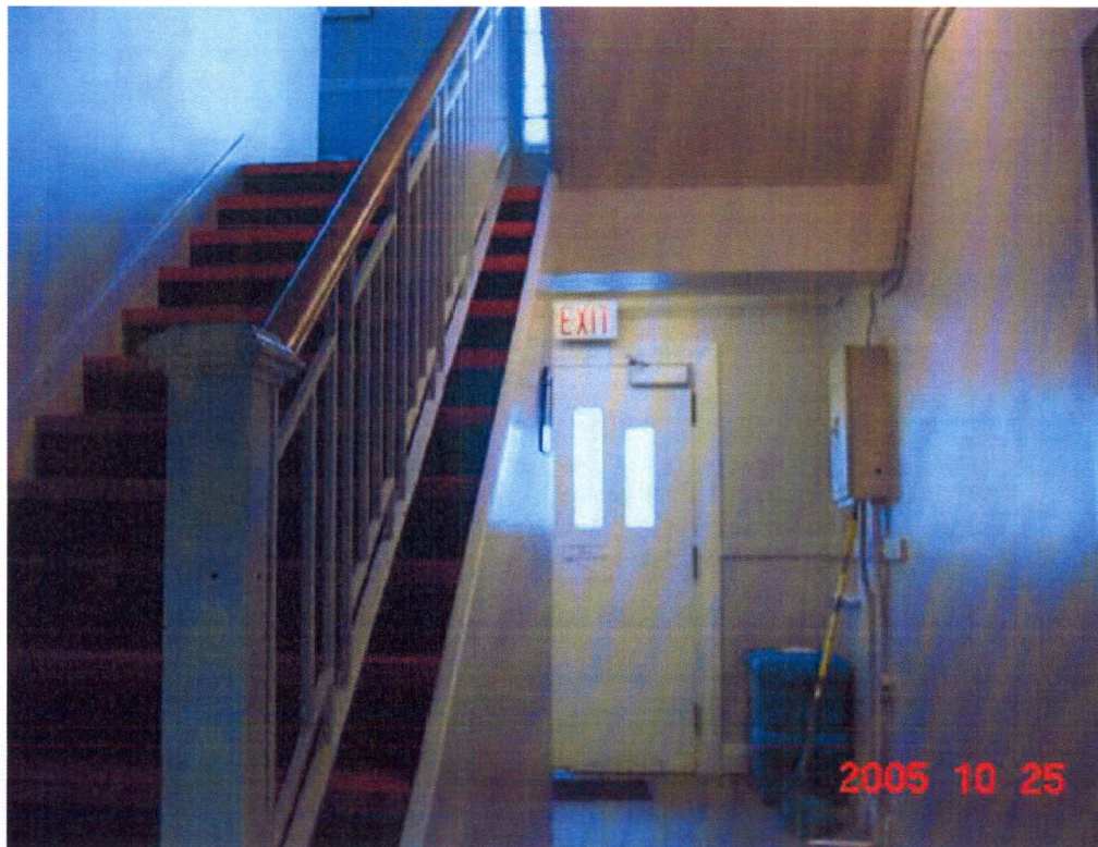
Figure 10. Staircase, WP1058, Work Point Barracks, CFB Esquimalt (DND, 2005).
