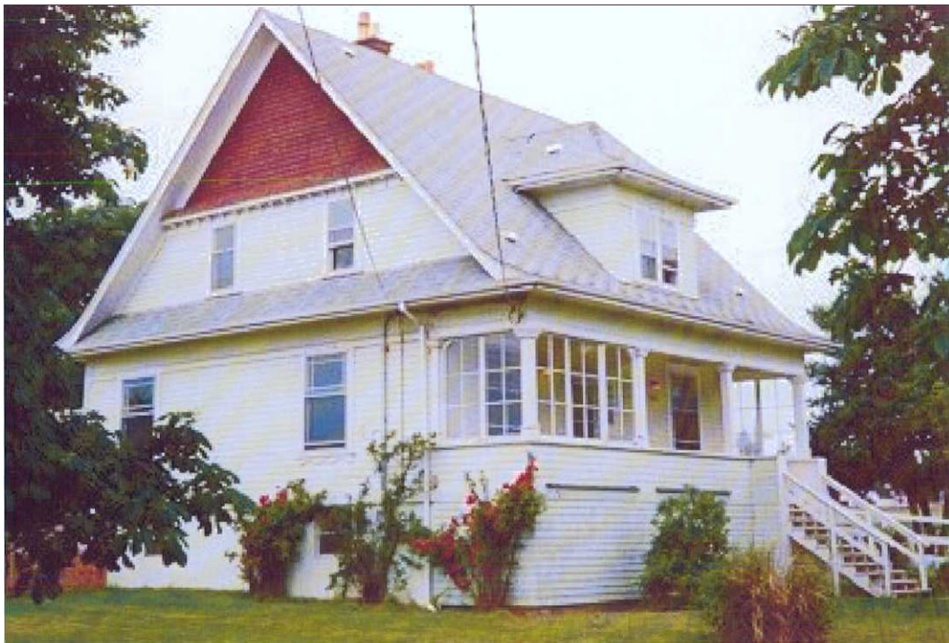
Figure 4. WP 1091 Ventures-NOTC Combined Barracks (DND, 2011).
