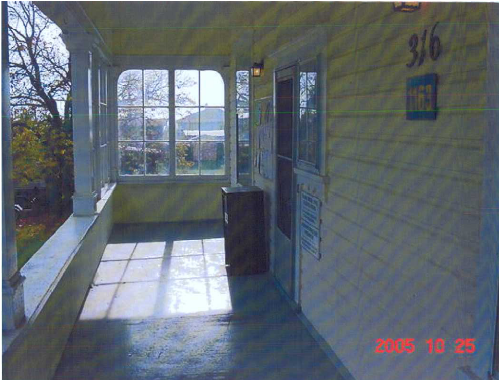
Figure 7. Front verandah, WP1163, Military Family Support Centre, Work Point Barracks, CFB Esquimalt (DND, 2011).
