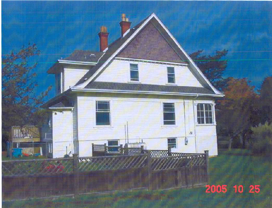
Figure 5. Side (south) elevation, WP 1163, Work Point Barracks, CFB Esquimalt (DND, 2011).
