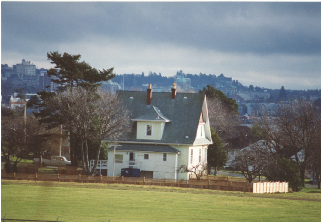
Figure 6. Rear elevation, WP 1163, Work Point Barracks, CFB Esquimalt (DND, 2011).
