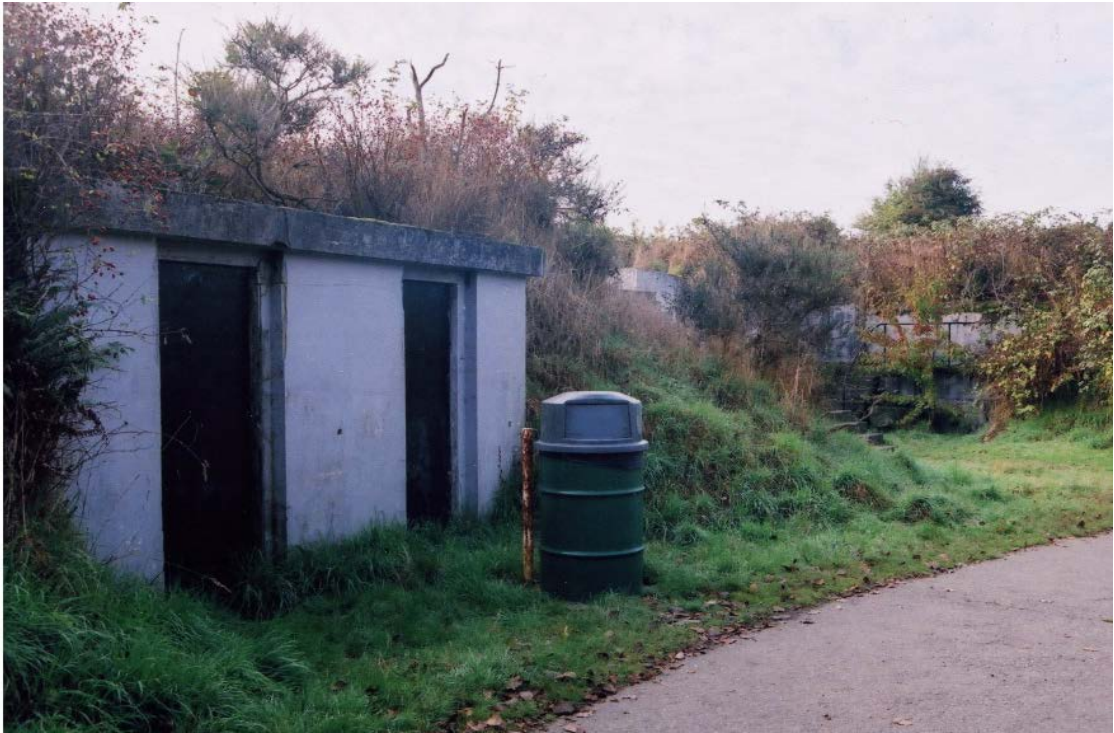
Figure 6. WP1191, right, with the underground passage toward WP1192 to the left (Ian Doull, Parks Canada, 2011).
