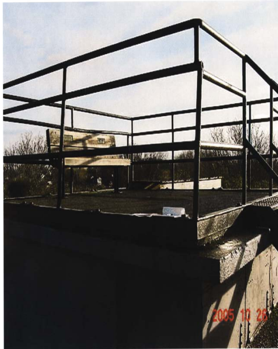
Figure 15. Roof of WP1192 with public park bench (DND, 2005).
