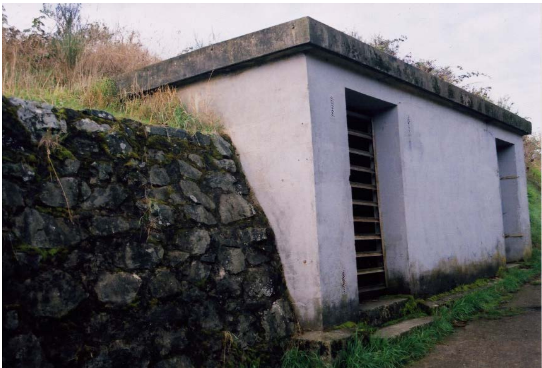
Figure 7. WP1191 with supporting wall, left (Ian Doull, Parks Canada, 2011).
