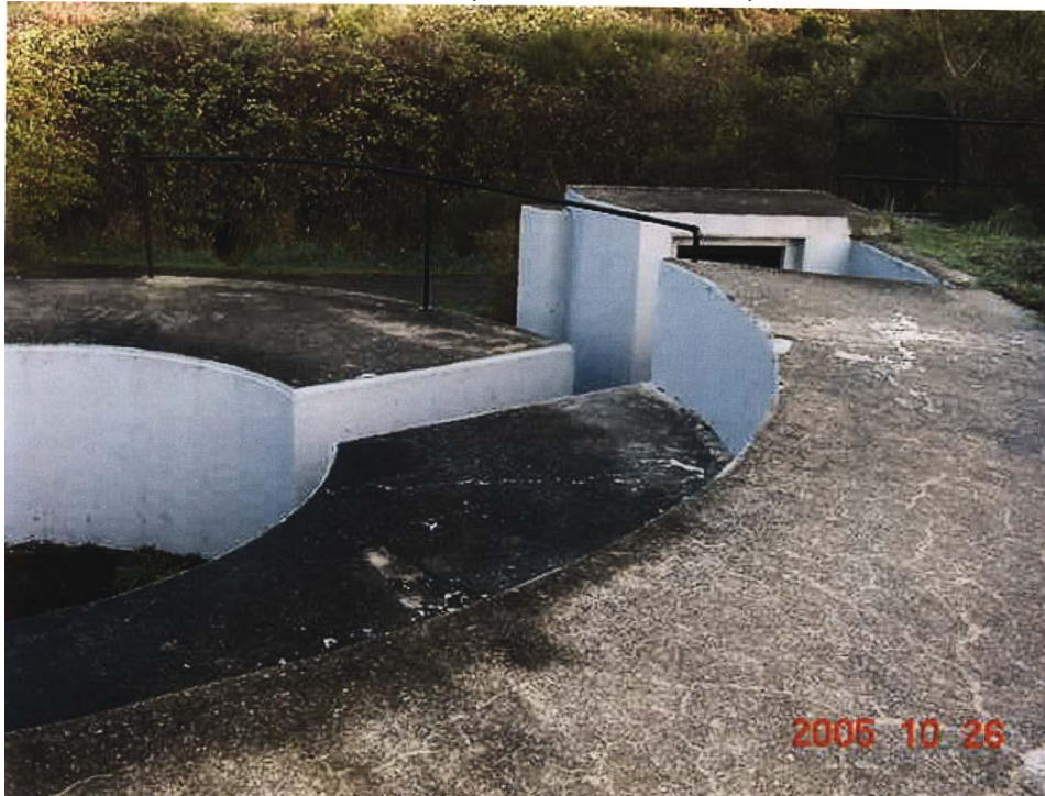
Figure 31. Annulus and parapet, WP1328, gun battery, Corps of Royal Engineers, constructed 1895, modified 1923/24 and 1938 (DND, 2006).
