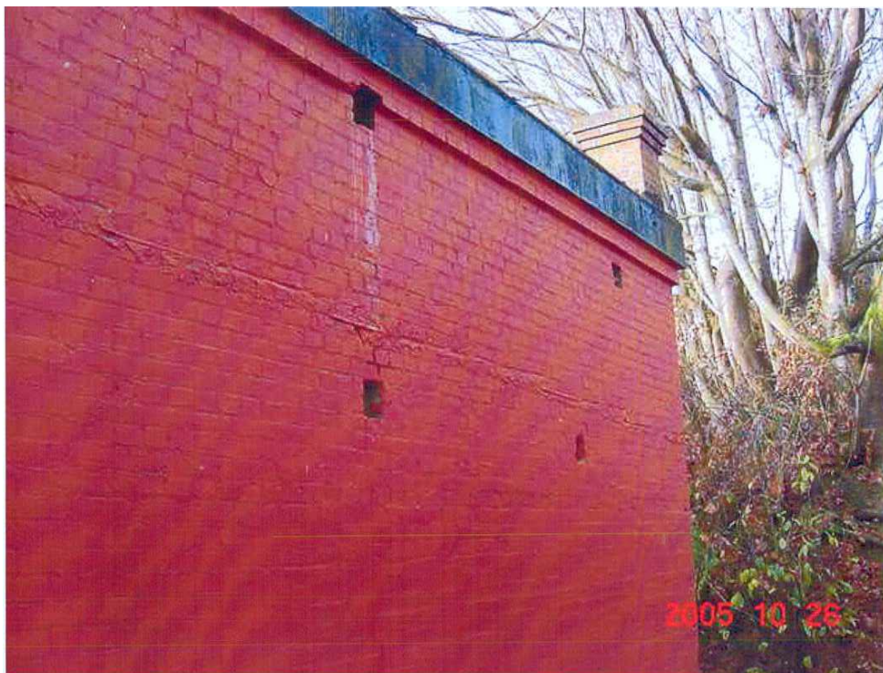
Figure 24. WP1199, north elevation (DND, 2005).
