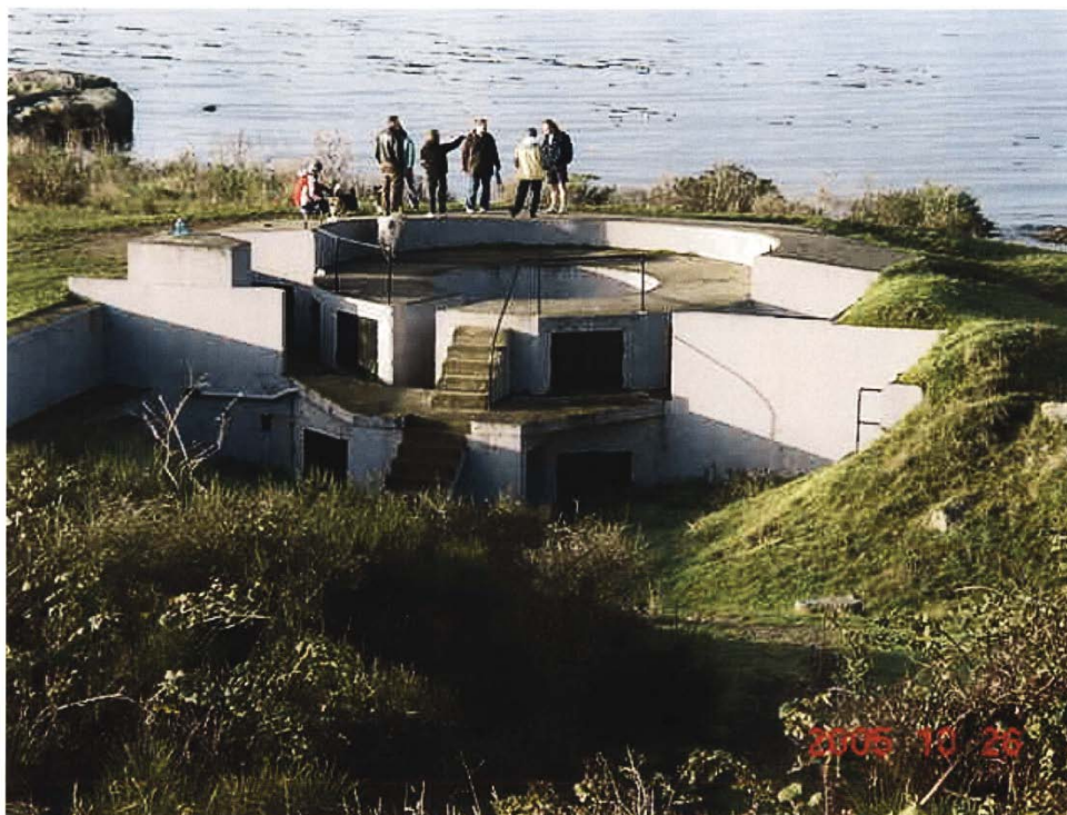
Figure 36. WP1329, gun battery, looking out to the Juan de Fuca Strait, Corps of Royal Engineers, constructed 1895, modified 1923/24 and 1938 by (DND, 2005).
