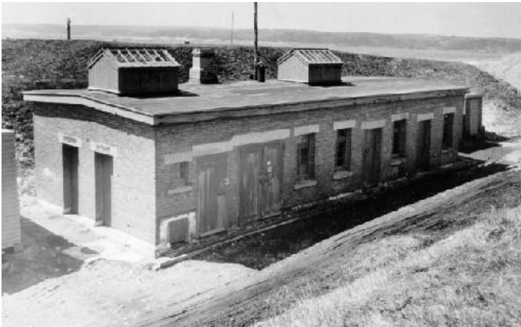
Figure 56. Comparative for WP1200, Oil Stores/Artificer's Shop, Fort McNab, Halifax, Nova Scotia, 1906, Royal Engineers (Parks Canada Agency, historicplaces.ca , accessed 29 January 2013). Scores: 15-0-6/9-8-4-2/4/11-5 = 64.
