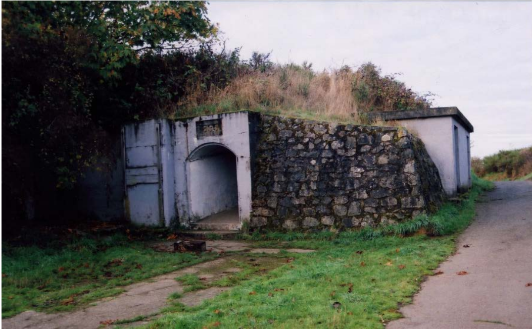
Figure 8. Opening to the underground passage from behind WP1191 to the former keep of Fort Macaulay (Ian Doull, Parks Canada, 2011).
