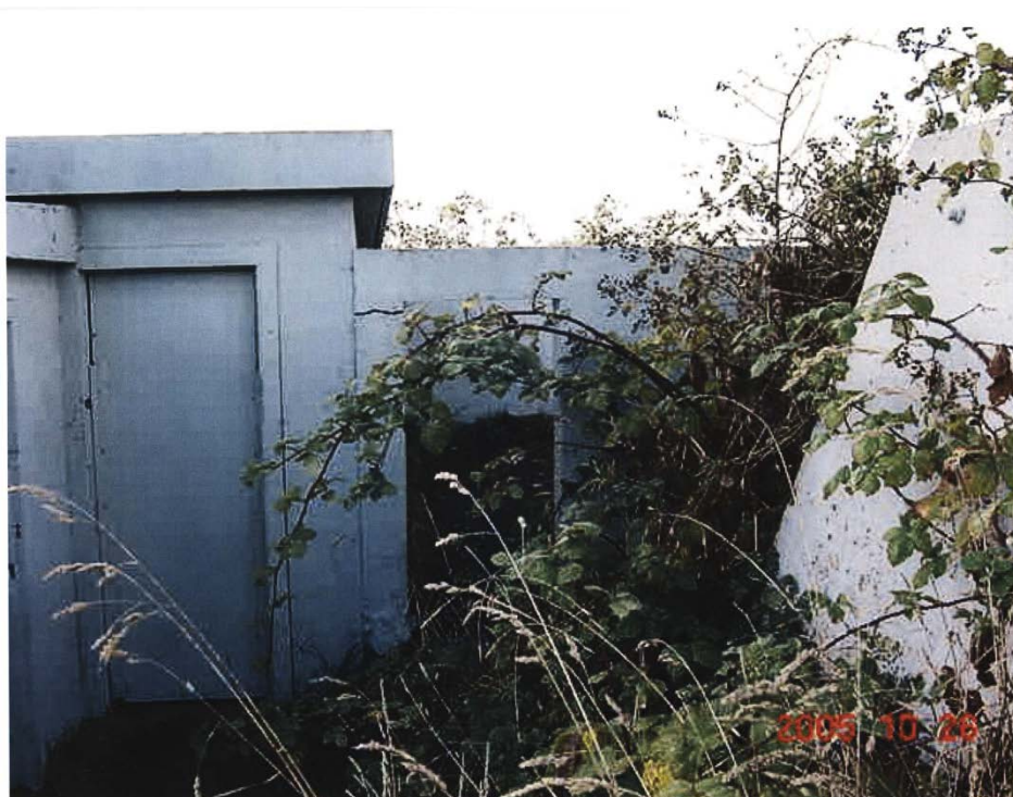
Figure 14. Entry to WP1192, Battery Command Post (DND, 2005).
