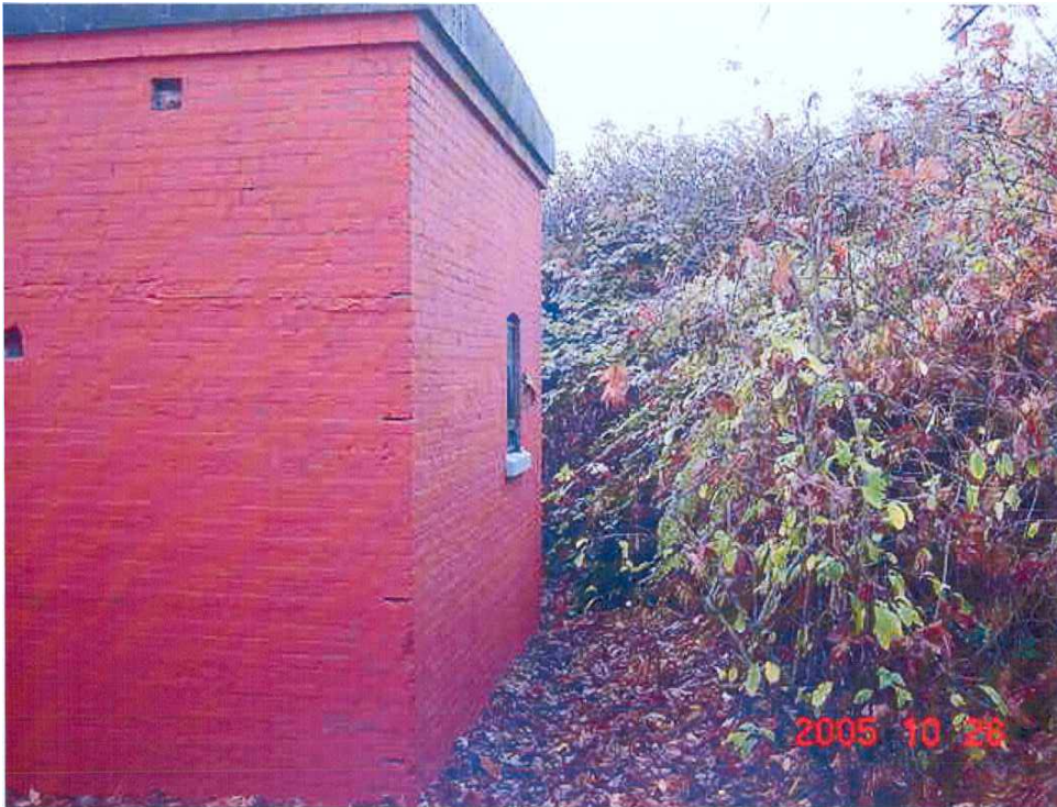
Figure 23. WP1199, east and north elevations (DND, 2005).
