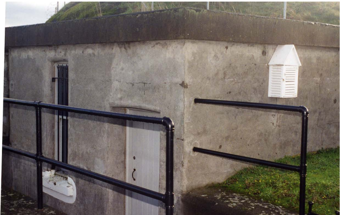
Figure 47. Fort Rodd Hill Artillery Store, 1903, Corps of Royal Engineers (Joan Mattie, Parks Canada, 1997).
