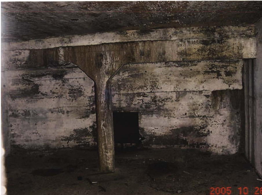
Figure 19. Interior, Crew Shelter WP1196 (DND 2005).
