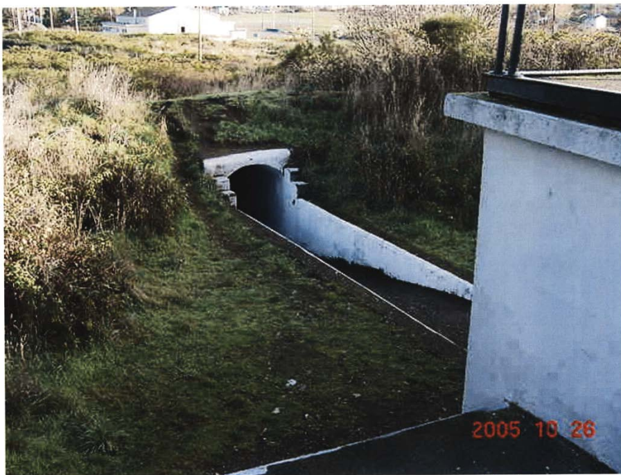
Figure 11. Entrance from the underground passageway to WP1192, right, in the former keep (DND 2005).
