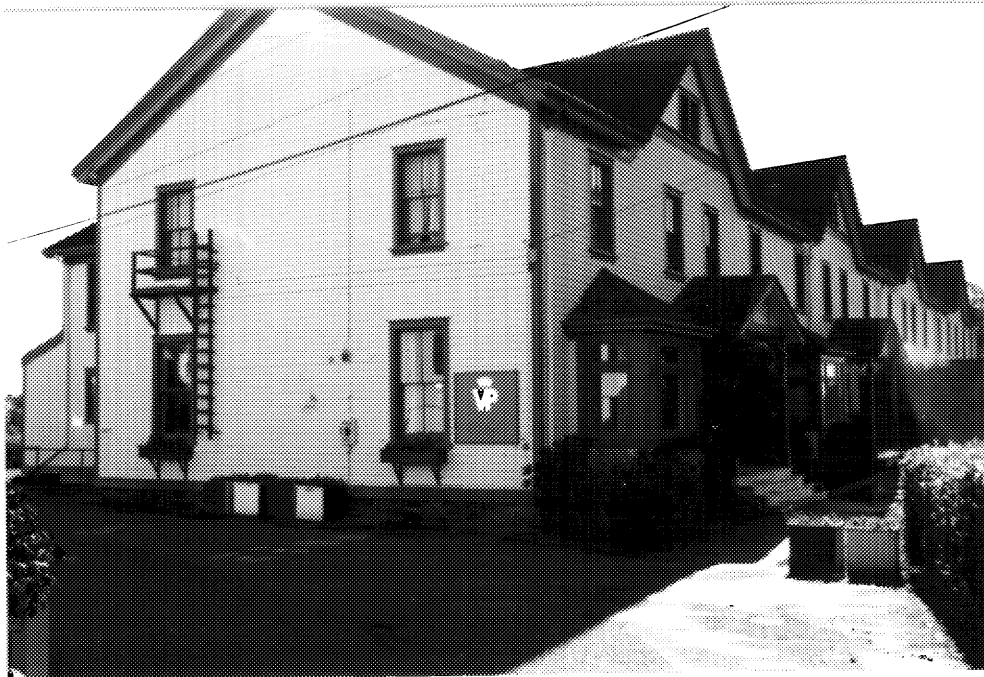
10 Officers' mess, side (west) and main (south) elevations. (Ian Doull, AHB, Parks, 1989.)
