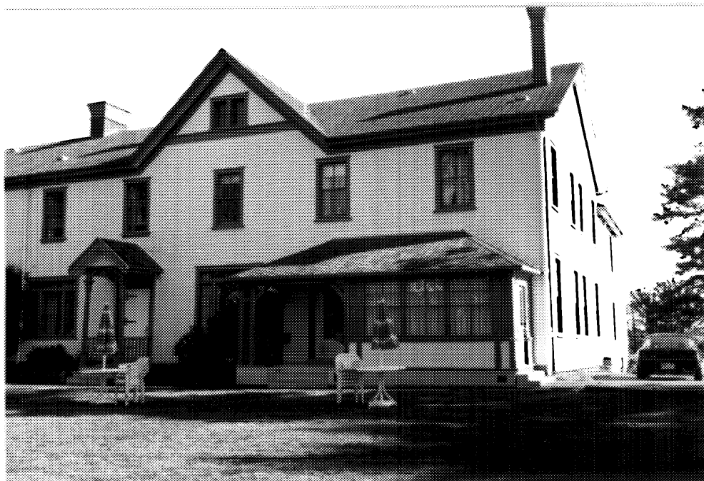
11 Officers' mess, main and side (east) elevations. (Ian Doull, AHB, Parks, 1989.)
