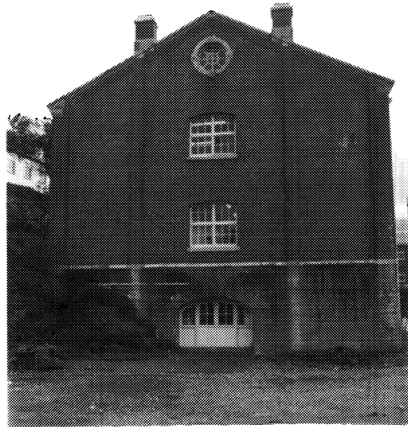
4. Details, north elevation of Warehouse D85. (DND)
