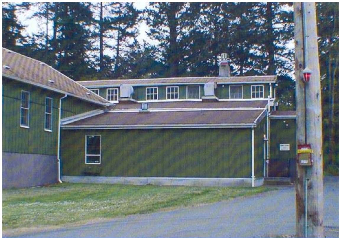
Figure 12. AH1015, Rear elevation, Kitchen Mess, Albert Head, 1940 (DND, 2011).
